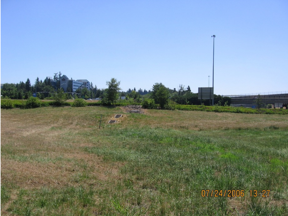
Photo 3: WQ Extended Dry Detention Pond looking south towards the outlet control structure.
