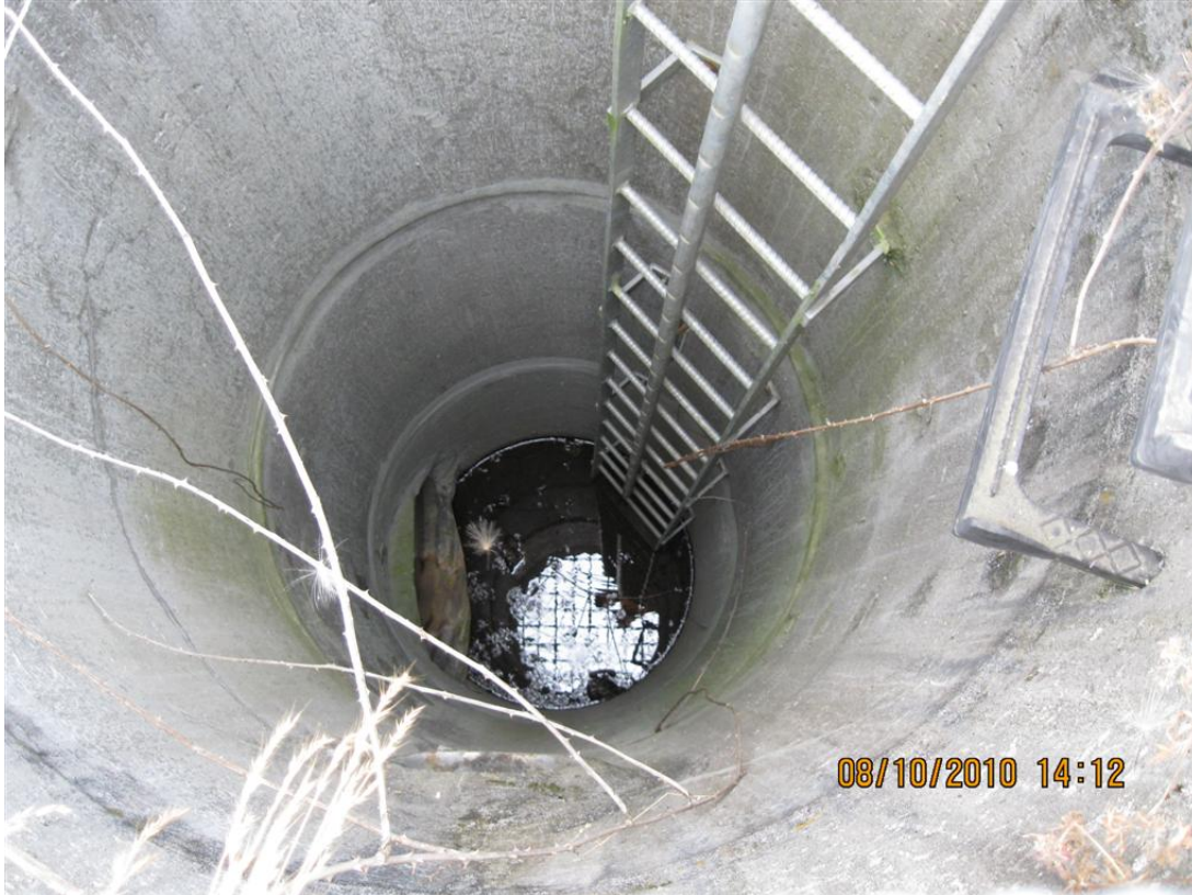
Photo 5: Special Manhole with emergency overflow grate looking down.
