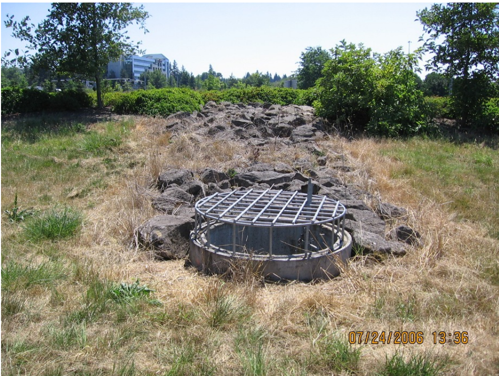
Photo 2: Emergency overflow grate with maintenance access rip rap pad behind.
