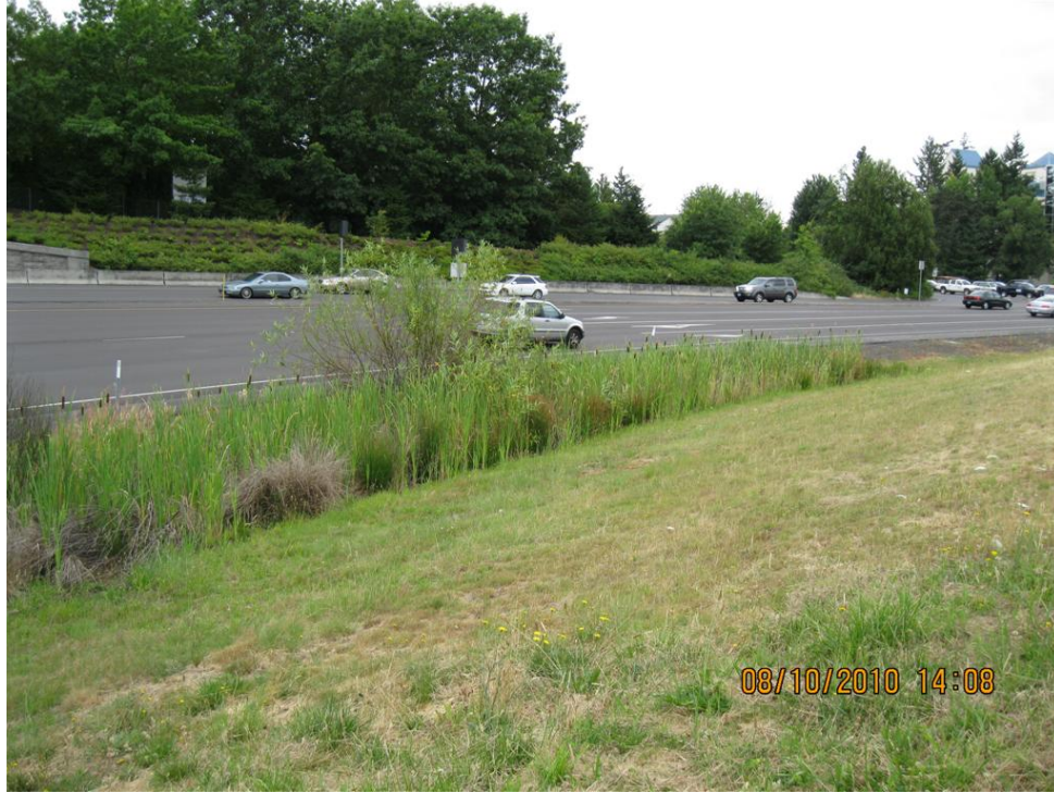
Photo 3: Center of WQ swale looking towards the south.
