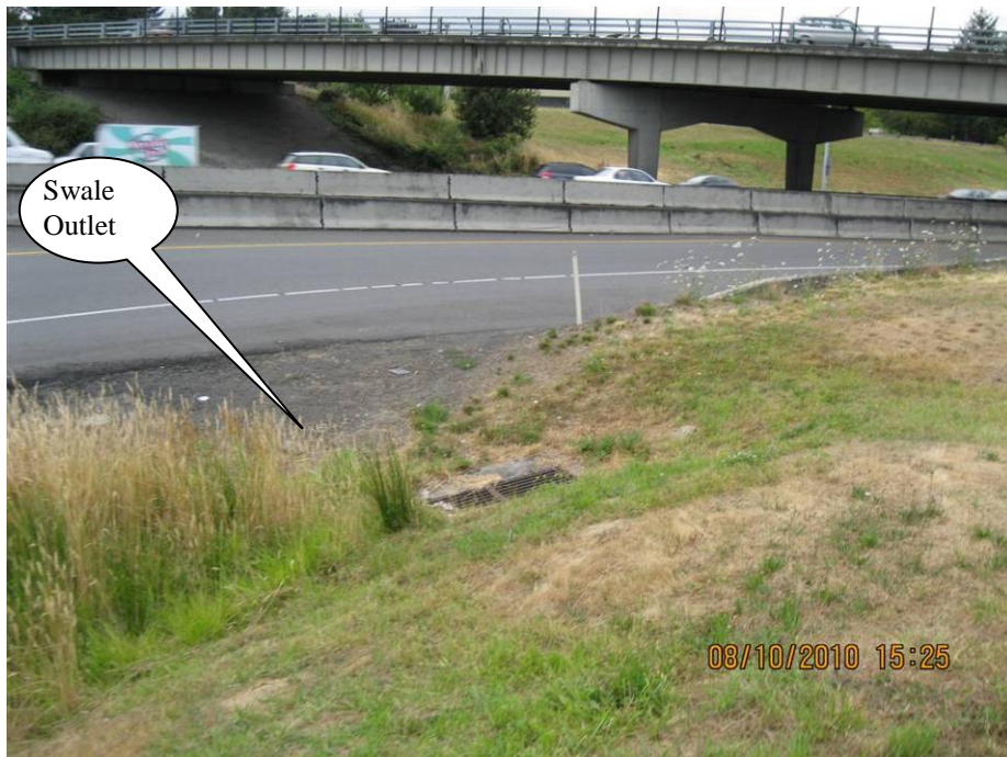
Photo 6: Outlet to WQ Swale looking south to southwest.
