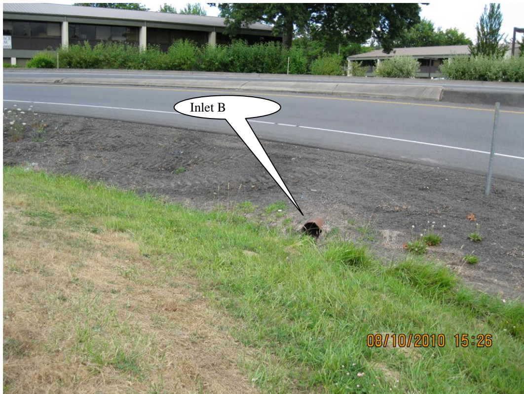
Photo 4: WQ Swale Inlet B at midpoint of swale.
