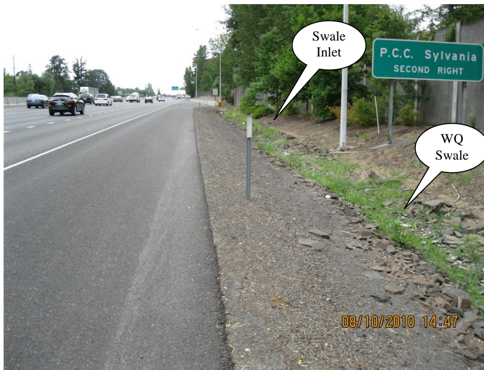
Photo 1: WQ Swale looking towards the north along the northbound travel lanes of I-5 (Hwy 001).
