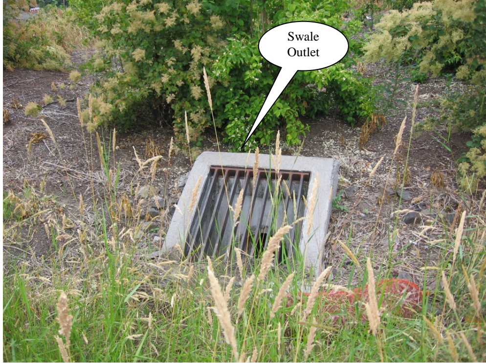
Photo 3: Ditch inlet serving as outlet for swale at eastern end of swale.
