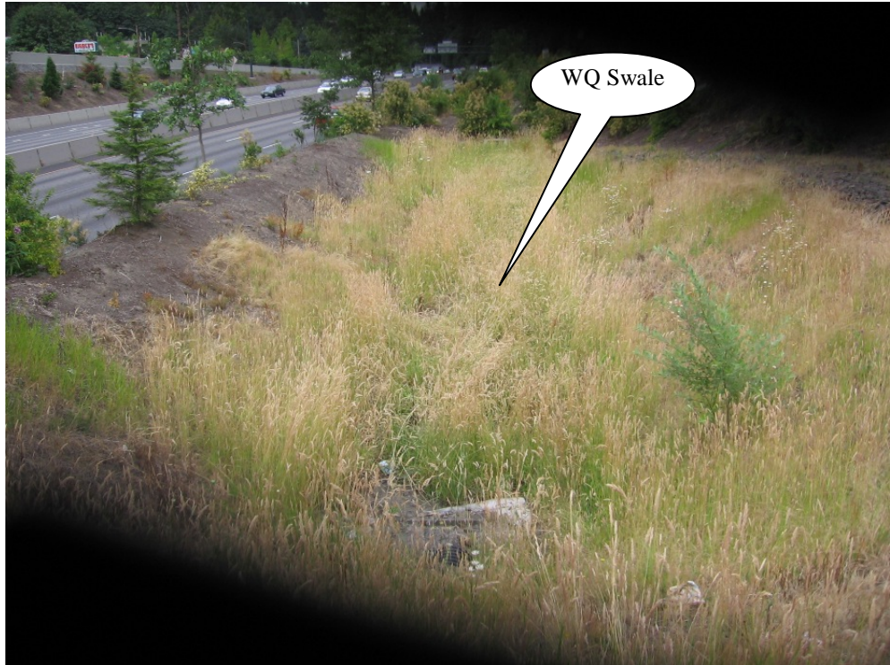
Photo 4: Looking west toward WQ Swale. US 26 (Hwy 047) located on the left.
