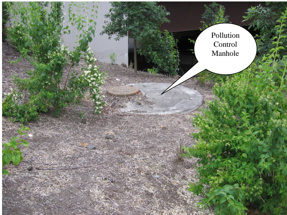
Photo 2: Looking west at Pollution Control Manhole; see point B, Operational Plan
