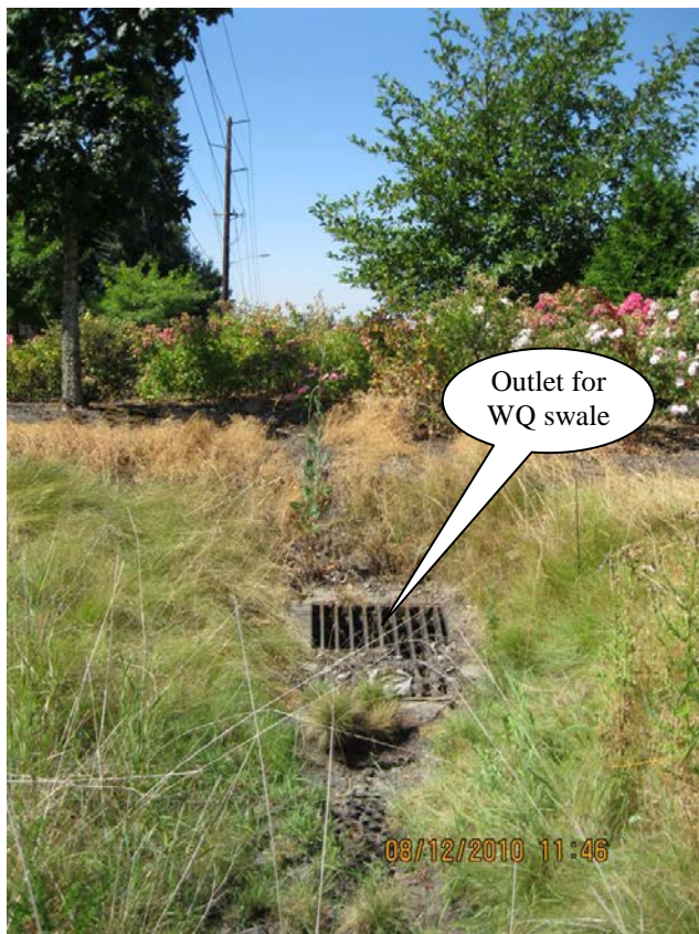
Photo 2: WQ swale outlet structure for the south swale.
