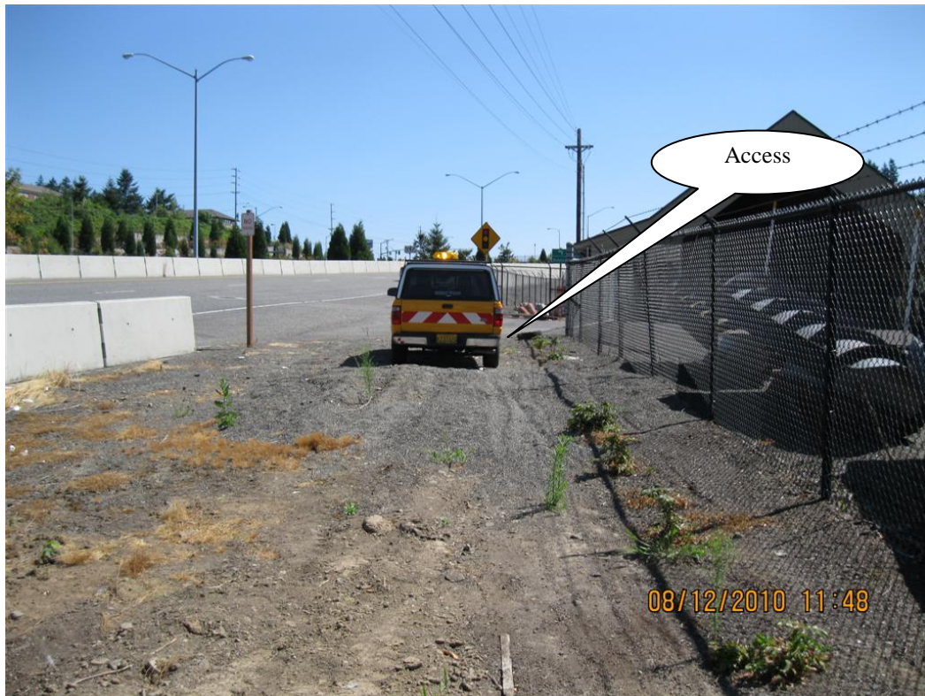
Photo 4: Access road from US 26 (Hwy 47) looking east. ODOT District Maintenance to the right.
