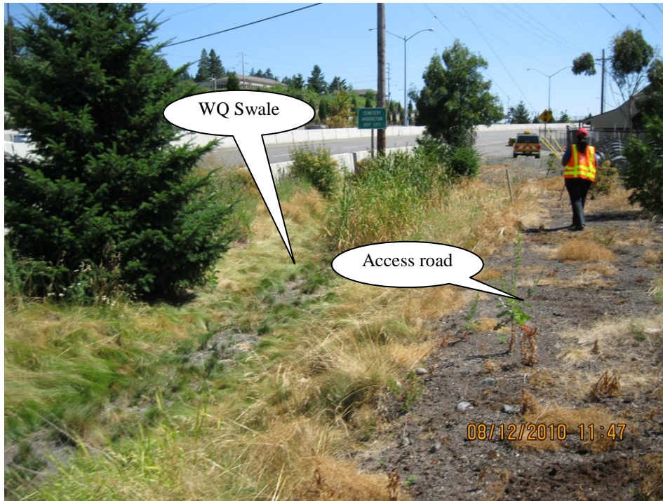
Photo 3: WQ swale outlet structure for the south swale.
