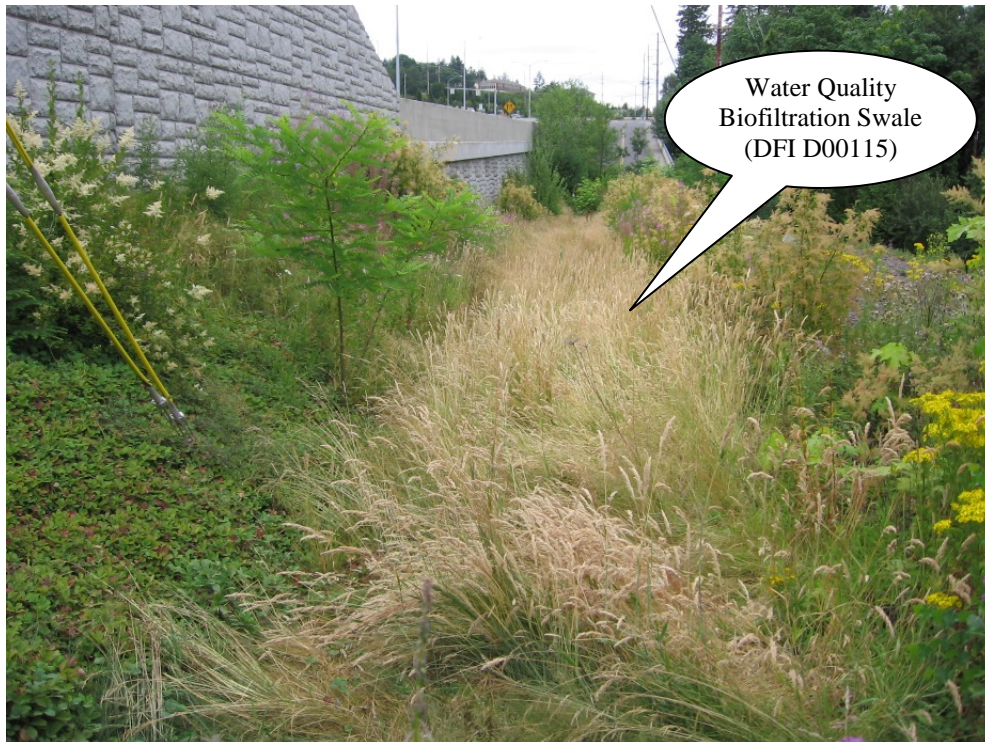
Photo 4: Overview of water quality biofiltration swale (DFI D00115.). Looking eastward with US26 (Hwy 047) behind the wall on the left.
