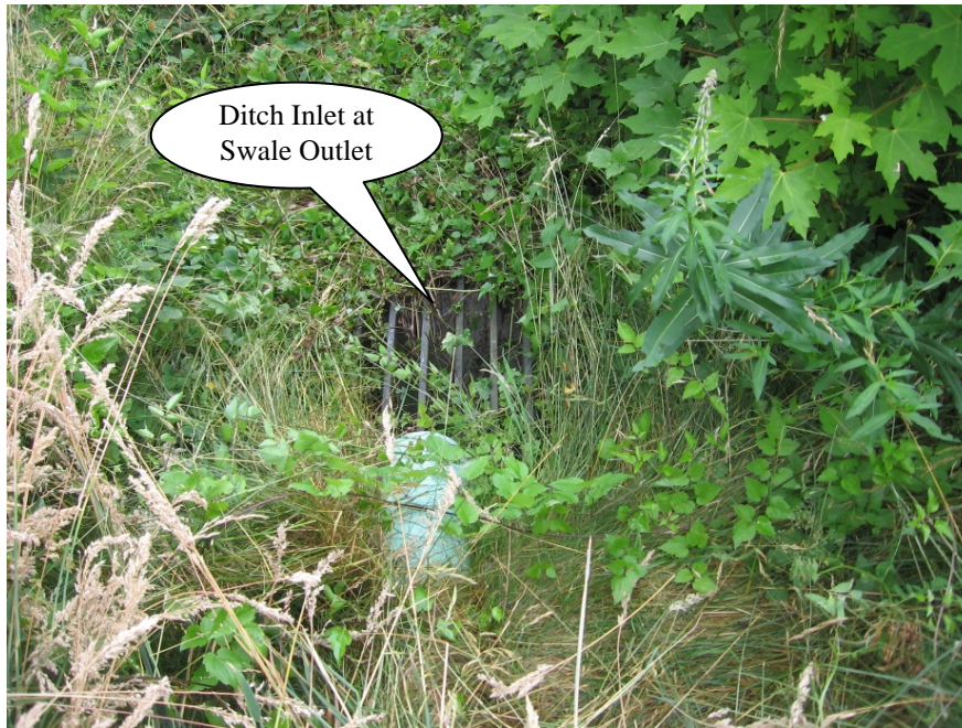
Photo 2: Ditch inlet at swale outlet.
