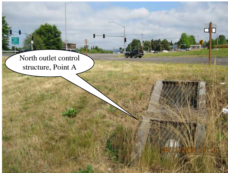
Photo 5: North outlet control structure, Point A, looking north.
