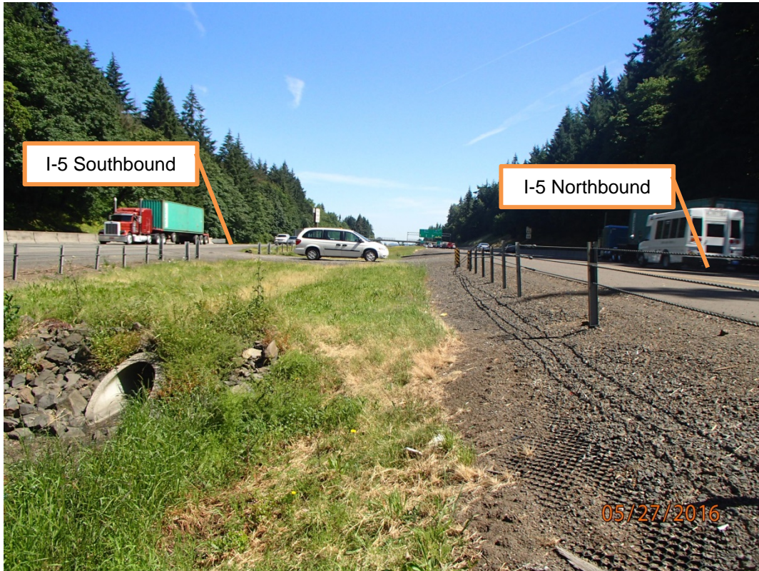
Figure 3: Facility access pad at inlet
