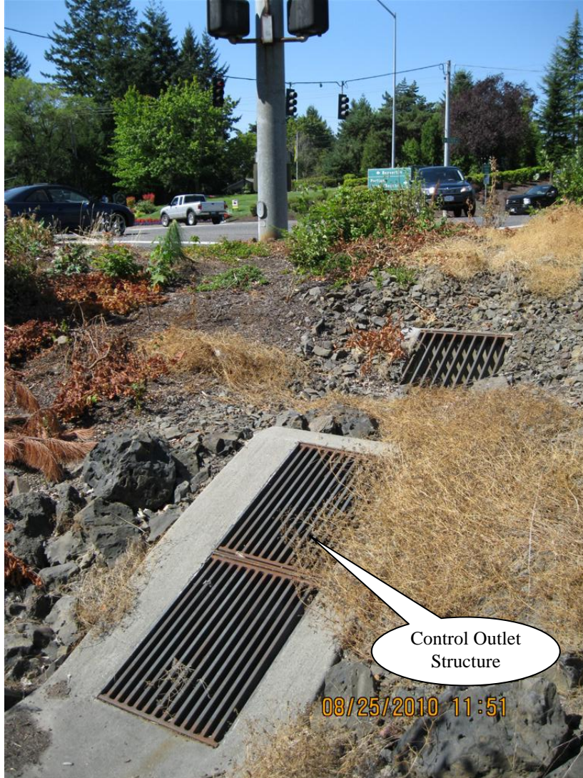
Photo 3: Control Outlet Structure to the Detention Pond; Point E, Ops Plan.
