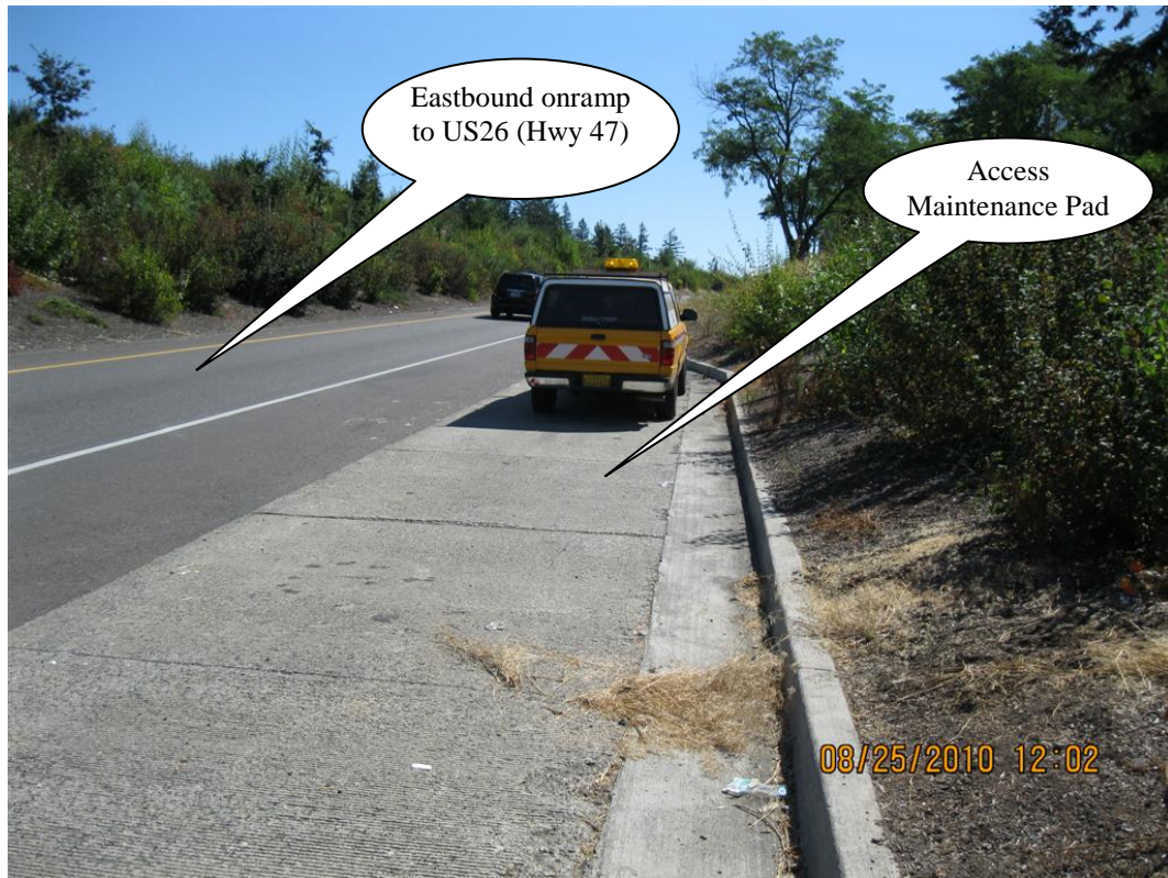
Photo 2: Access maintenance pad on eastbound onramp to US 26 (Hwy 47) looking east.
