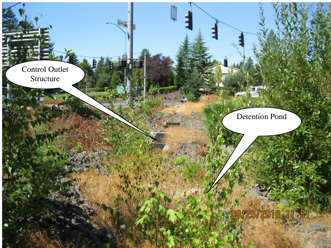
Photo 1: Detention pond facility looking west towards Cedar Hills Blvd. The riprap in the bottom of the pond forms a low-flow channel.
