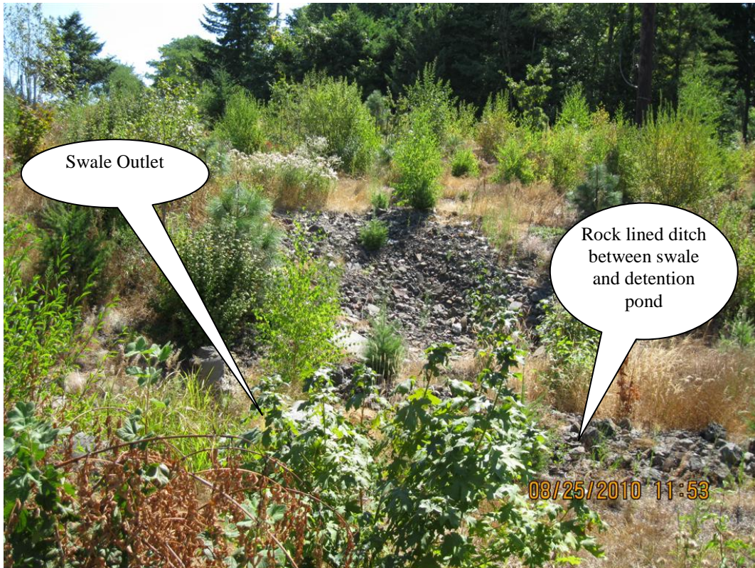
Photo 1: Looking east at the water quality biofiltration swale.
