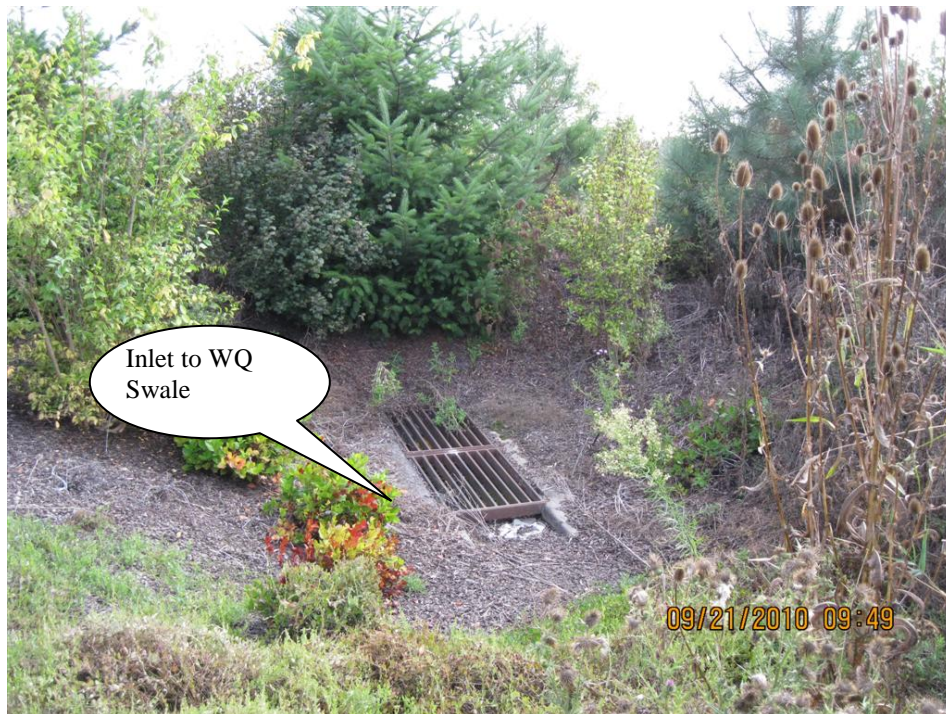
Photo 6: Outlet from extended detention dry pond at modified inlet. The two 8-inch drain pipes discharge into this structure which serves as the inlet for the nearby WQ biofiltration swale (DFI D00129), (Point E, Operational Plan)
