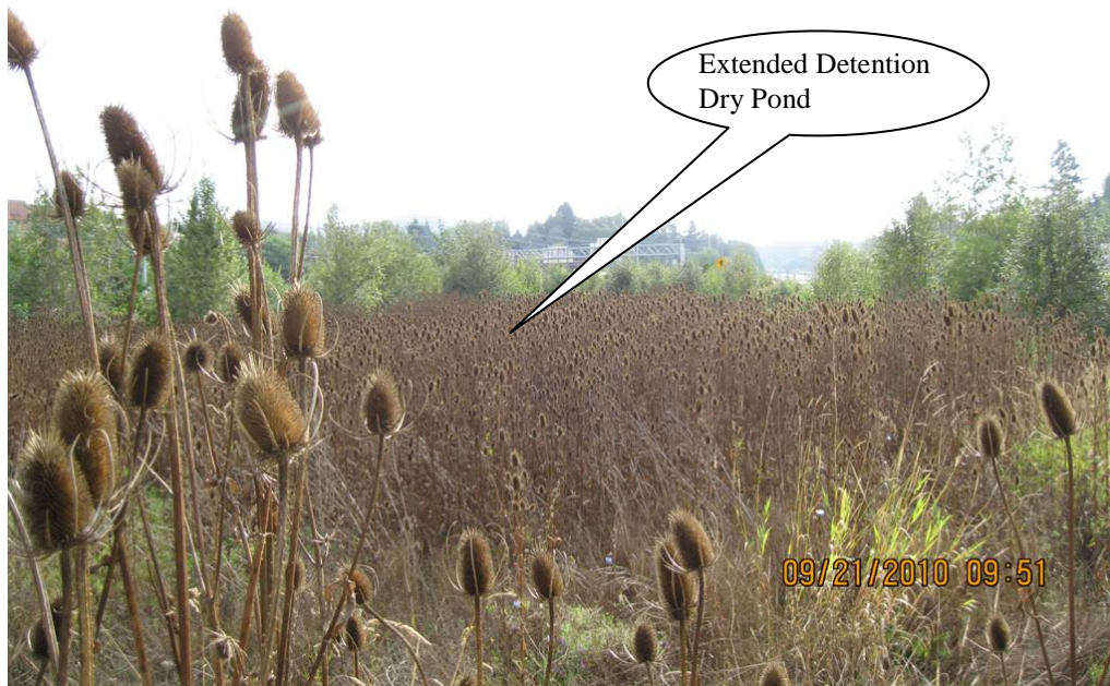
Photo 1: Extended detention dry pond looking northeast. Note the heavy vegetation with cattails.
