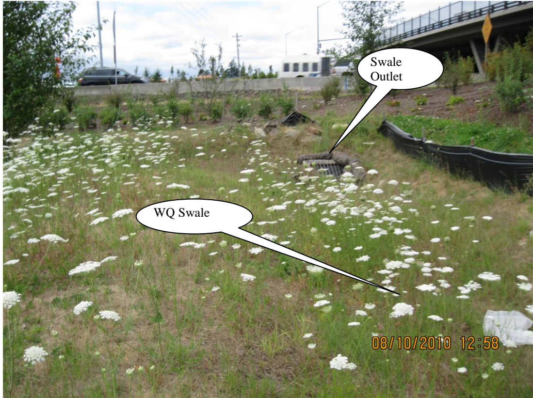
Photo 2: WQ Biofiltration Swale looking west. I-5 is located in the background.
