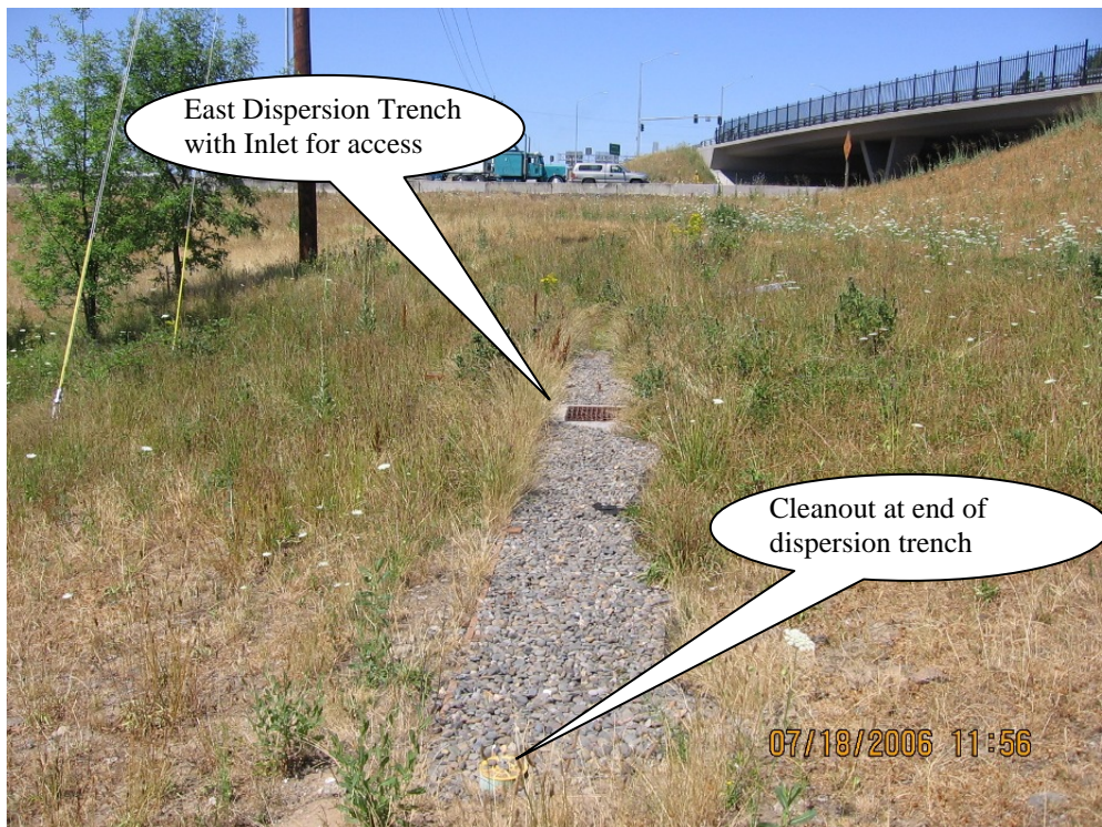
Photo 3: East Dispersion Trench, looking west. Interstate 5 is the background.
