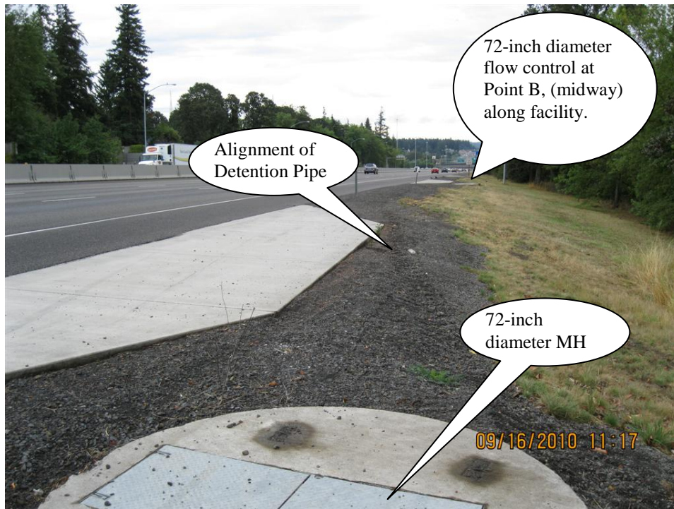
Photo 1: 20-foot deep inlet manhole at upstream end of detention tank/pipe facility.
