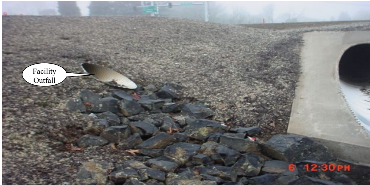
Photo 5: Facility Outlet (Taken December 2011)
