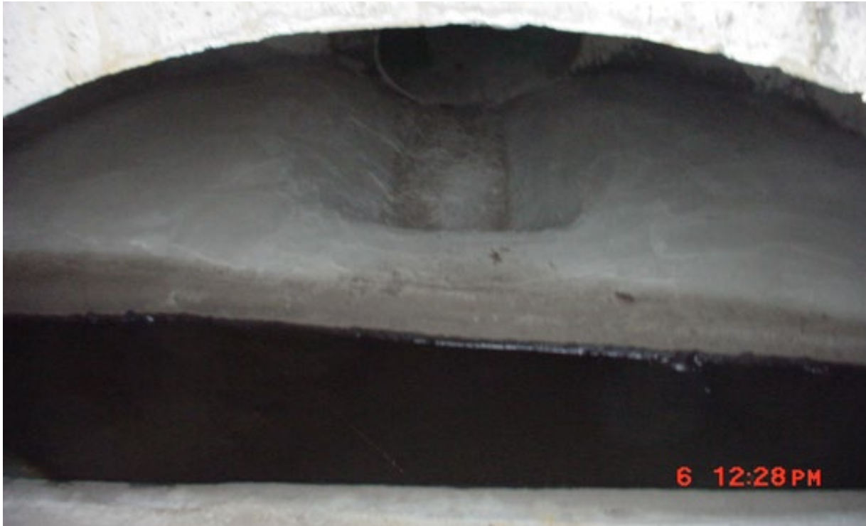
Photo 3: Diversion Manhole Weir (Taken December 2011)
