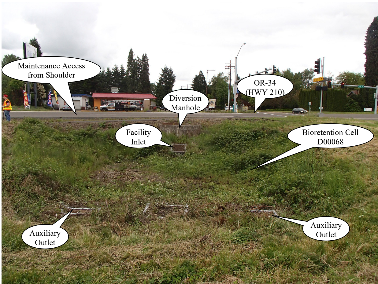
Photo 1 Facility Footprint (a) Looking South or Upstream (taken April 2016)
