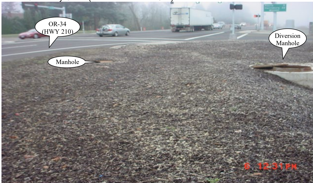
Photo 5: Embankment Slopes near Facility or Decreasing Mileage (Take December 2011)
