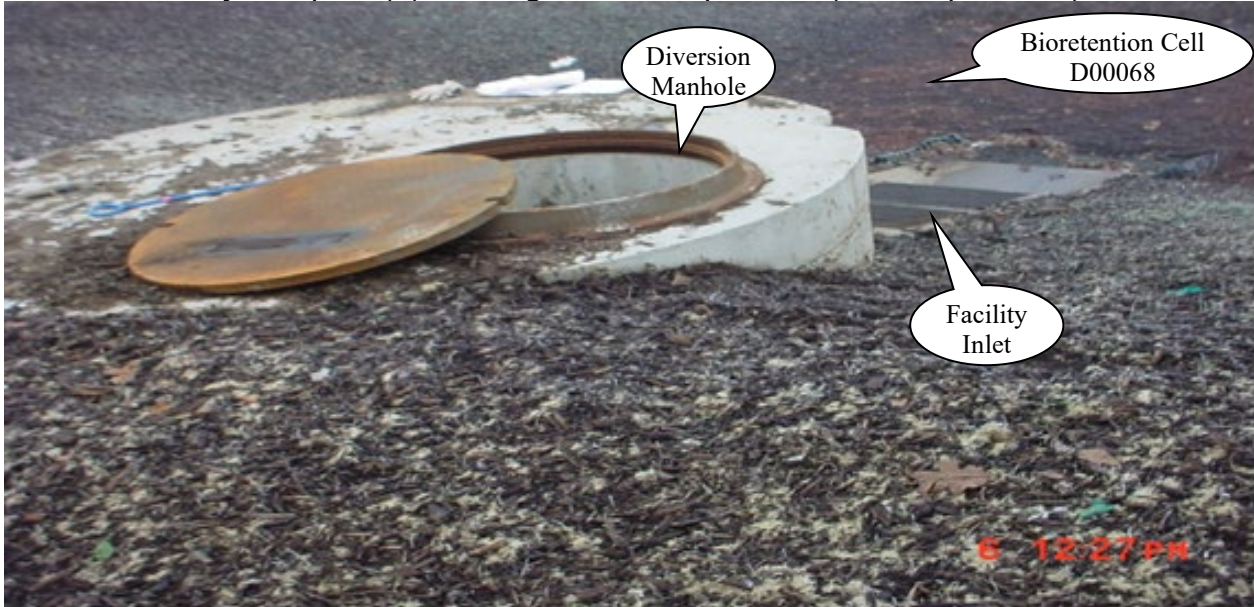
Photo 2: Diversion Manhole, Facility Inlet Looking North or Downstream (taken April 2016)
