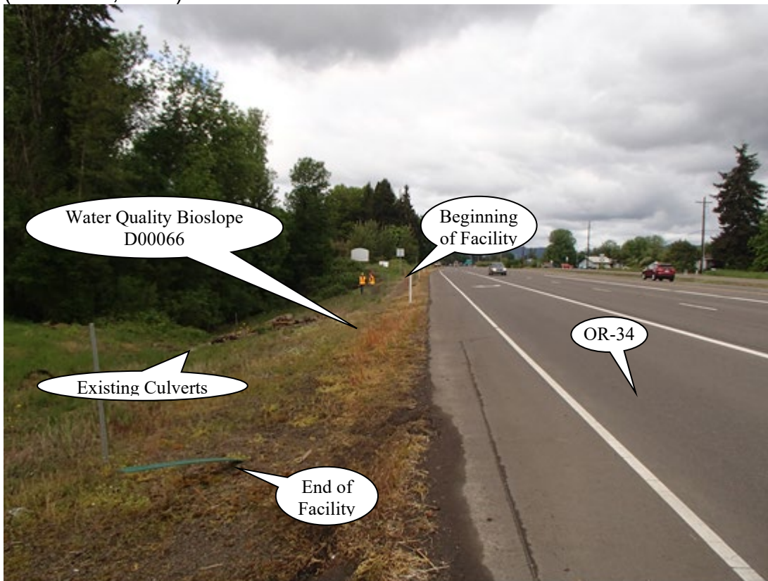
Photo 2: Facility Footprint (b) Looking from East or Decreasing Mileage (taken April, 2016)
