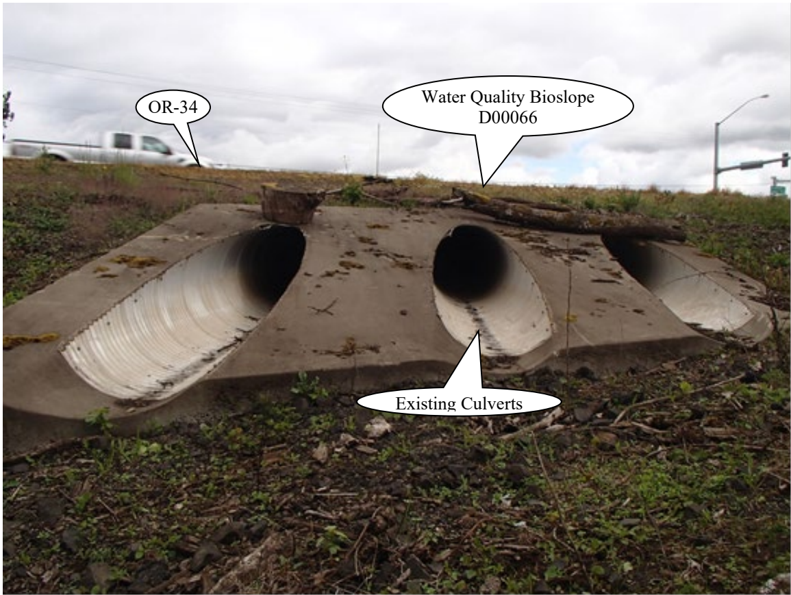
Photo 5: Existing Culverts Looking from South (taken April 2016)
