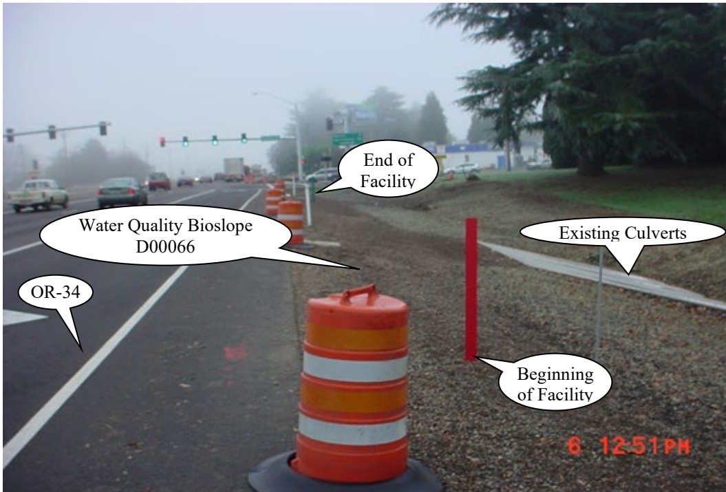
Photo 3: Facility Footprint (b) Looking from West or Increasing Mileage (taken Dec, 2011)
