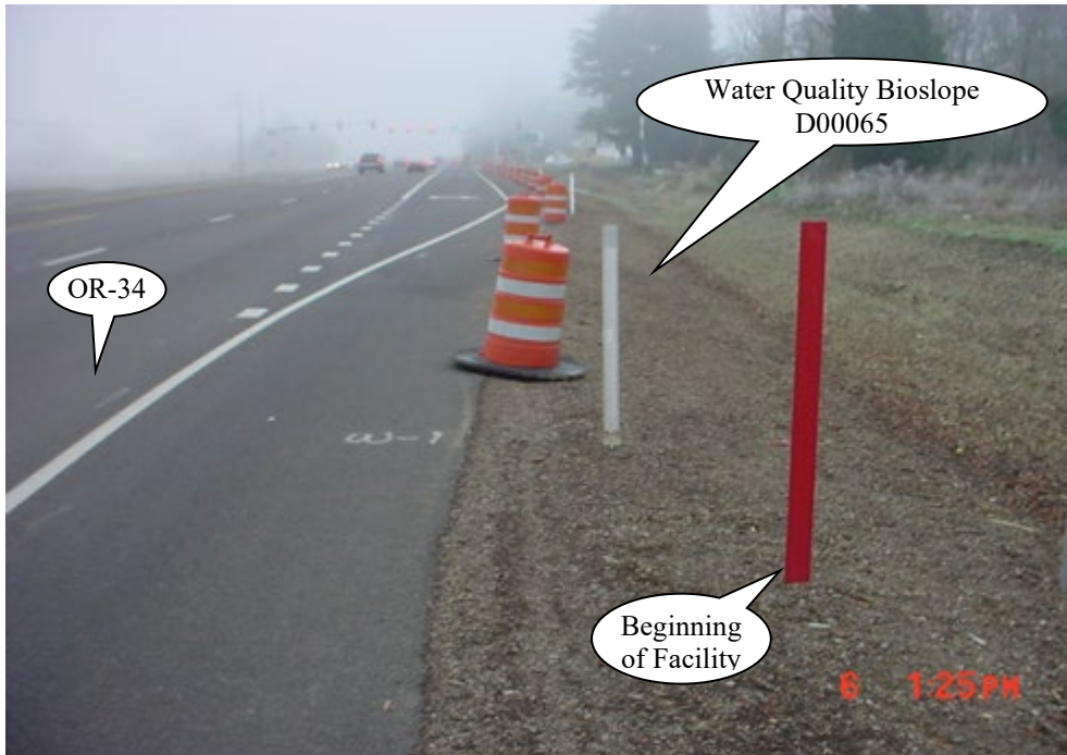
Photo 3: Facility Footprint (c) Looking from West or Increasing Mileage (taken Dec, 2011)
