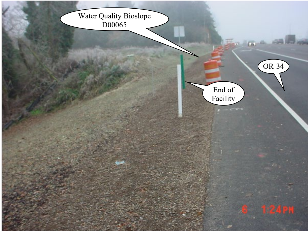
Photo 1: Facility Footprint (a) Looking from East or Decreasing Mileage (taken Dec, 2011)
