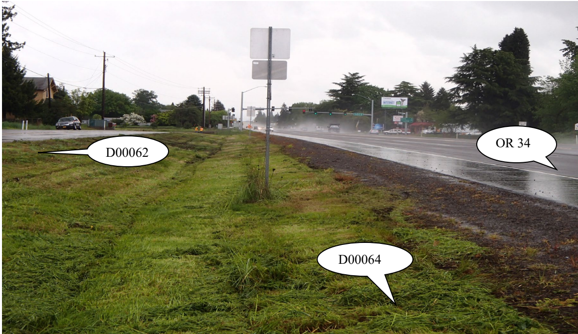
Photo 4: Facility foot print looking east, taken in 2016
