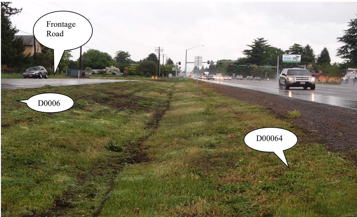
Photo 5: Facility foot print looking east, taken in 2016
