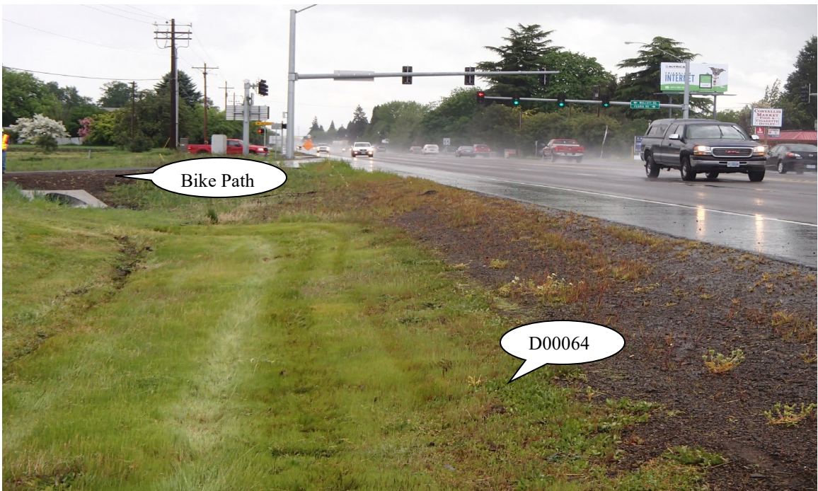
Photo 7: Facility footprint looking east, taken in 2016
