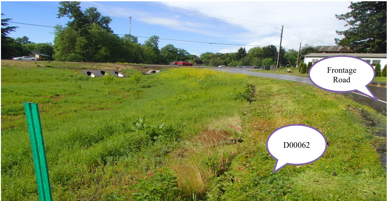
Photo 9: Surrounding culverts looking west, taken in 2016
