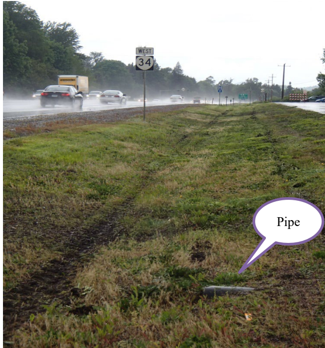
Photo 10: Pipe under facility looking west, take in 2016
