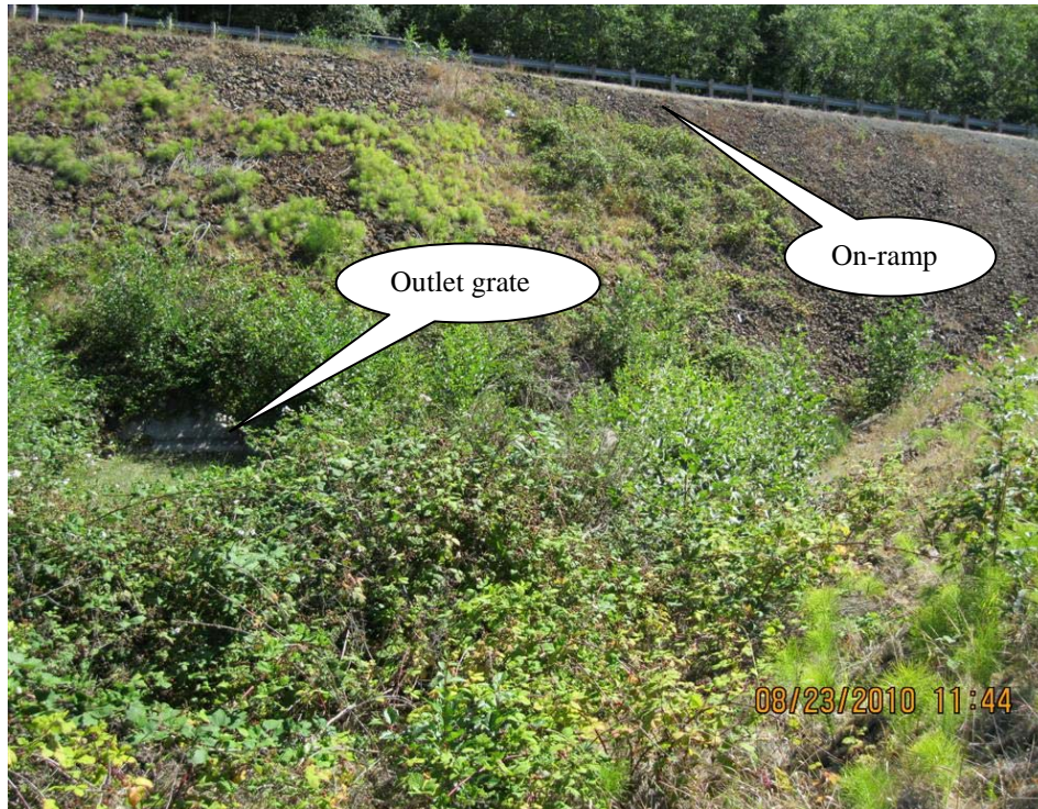
Photo 3: Outlet grate covered by vegetation
