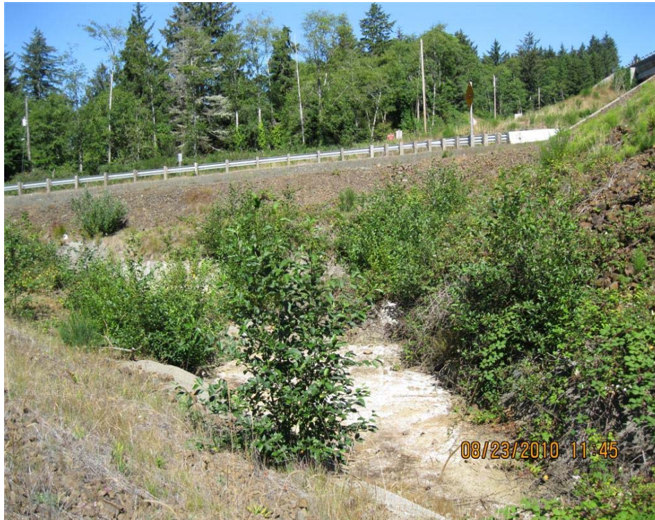
Photo 2: View of the detention pond facing north.
