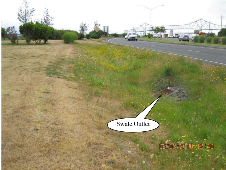
Photo 3: Midpoint of swale where swale outlet is obtained from ditch inlet.
