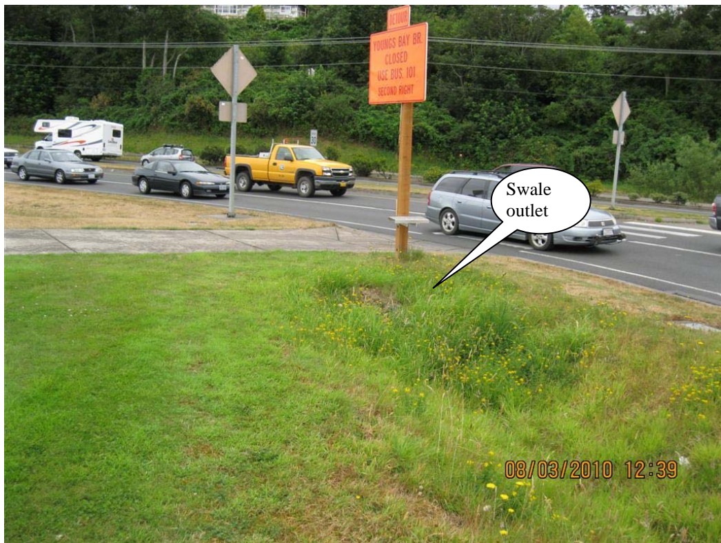
Photo 2: Swale outlet which is a 12-inch culvert that discharges in DFI D00054.
