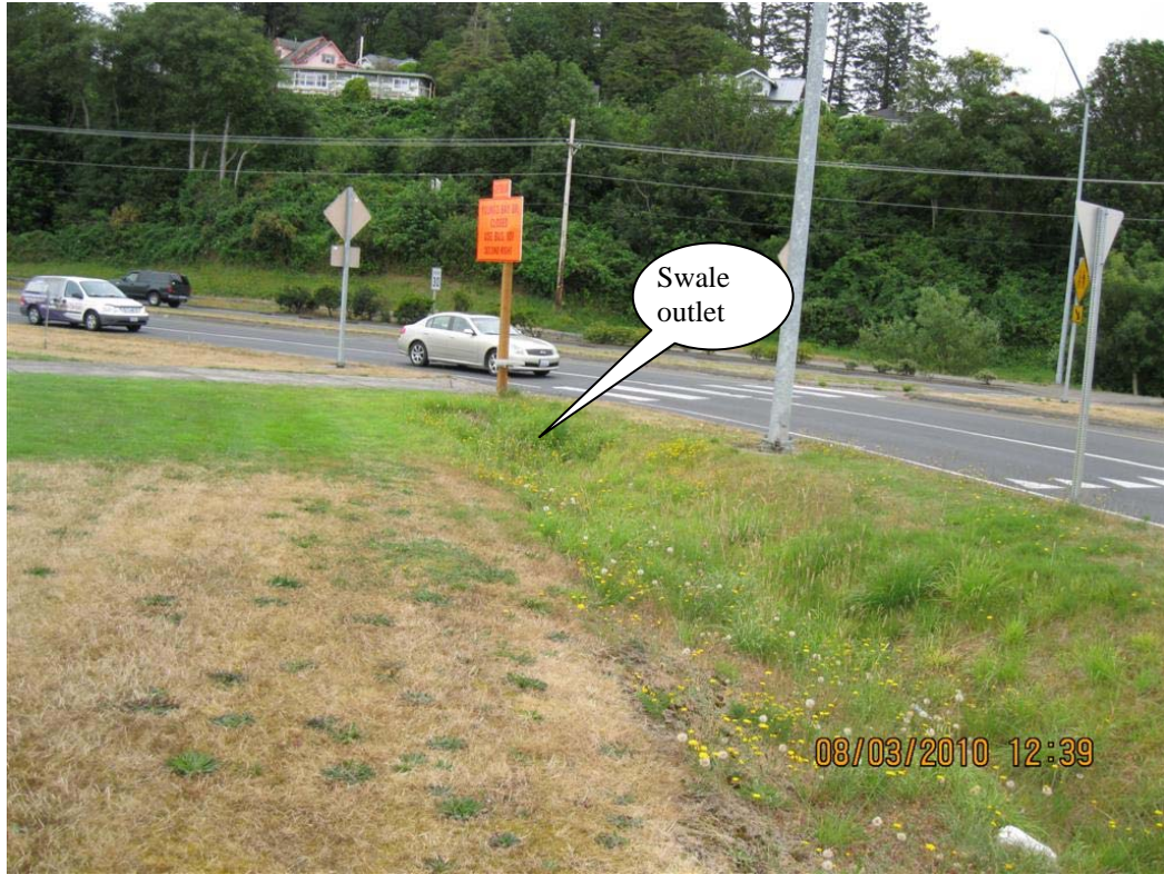
Photo 1: The swale looking east towards US 101. The swale outlet is a 12-inch culvert pipe.
