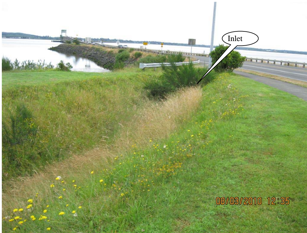
Photo 1: Looking towards the west to south-west at the swale inlet.
