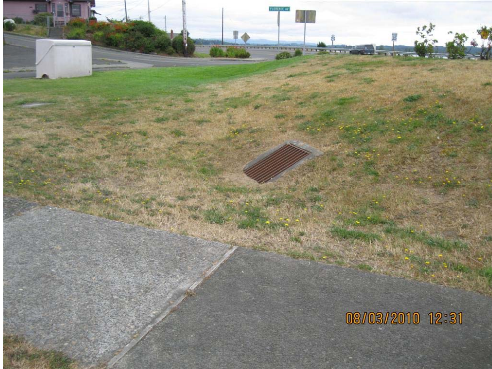
Photo 5: Ditch Inlet south of pump station. This inlet was originally to be end of swale.
