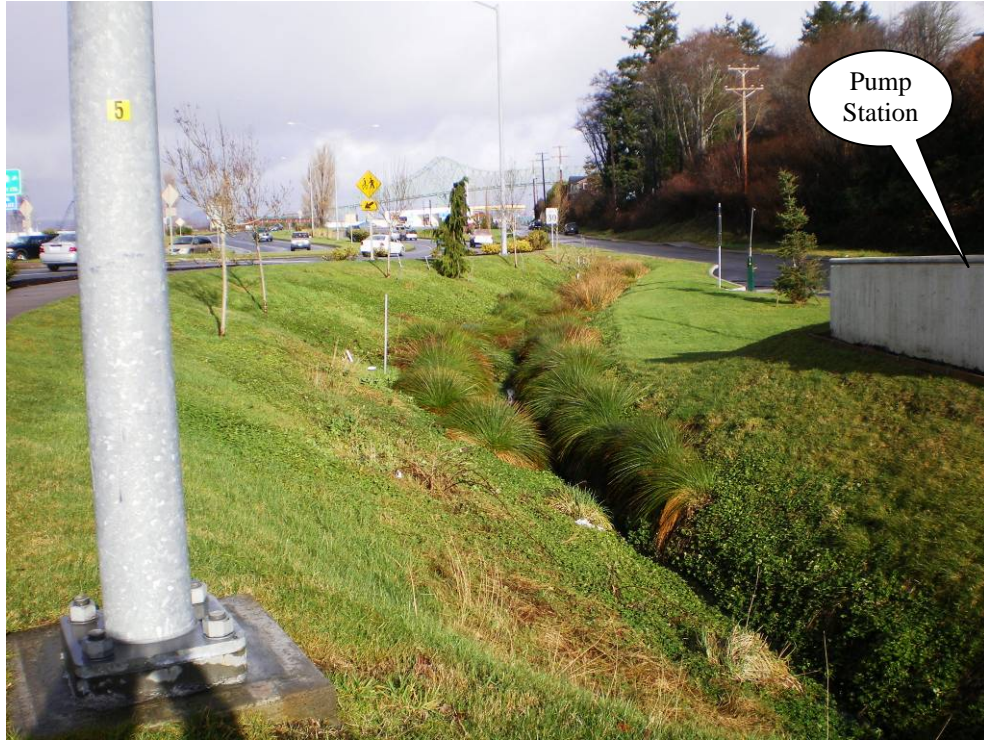
Photo 3: Swale looking towards the north from the pump station.
