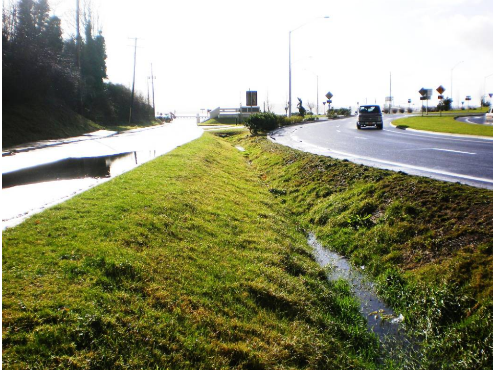
Photo 3: Swale looking south from middle of swale.
