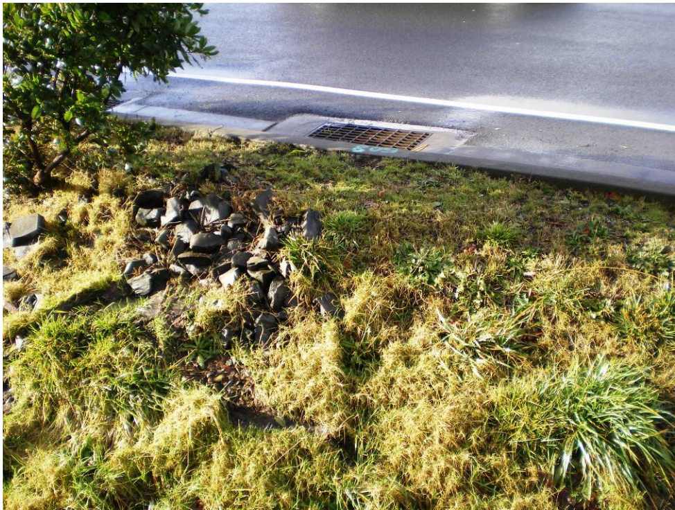
Photo 4: Sag inlet discharges directly into swale (Point D).
