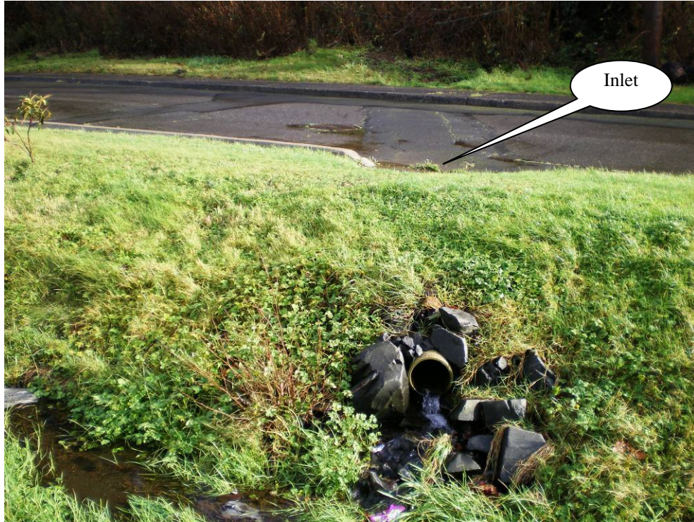
Photo 5: 12-inch inlet (Inlet C, Point C) draining into swale near midpoint.
