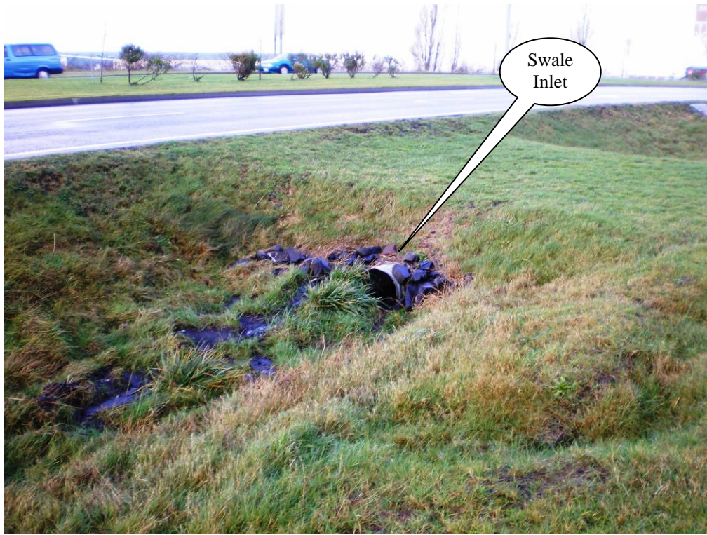
Photo 1: Swale Inlets at north end of swale looking north.
