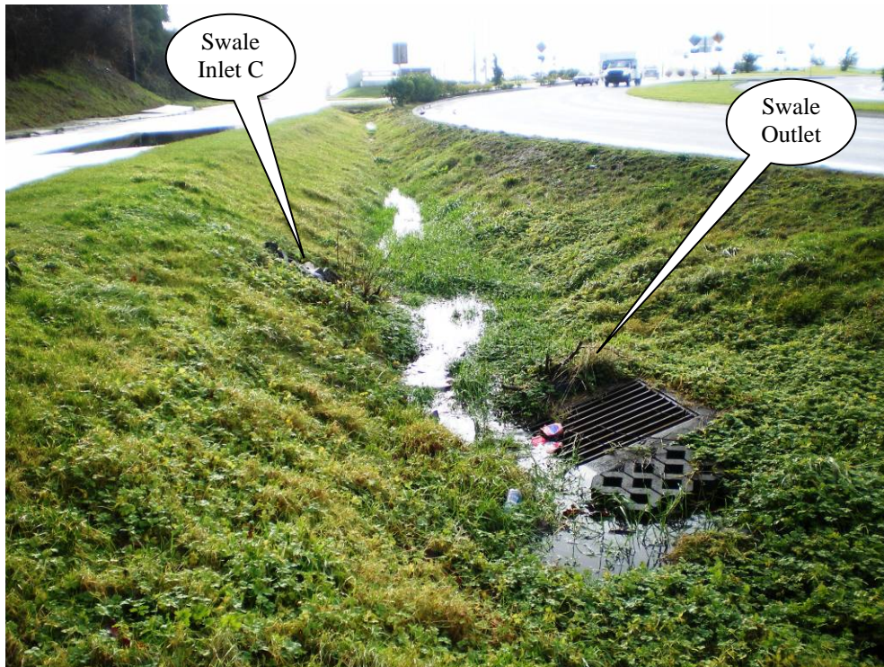
Photo 6: Swale outlet (ditch inlet) in middle of swale (Point F).
