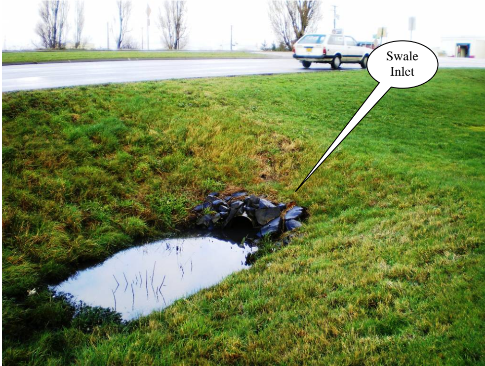
Photo 1: Swale Inlet at north end of swale looking north.
