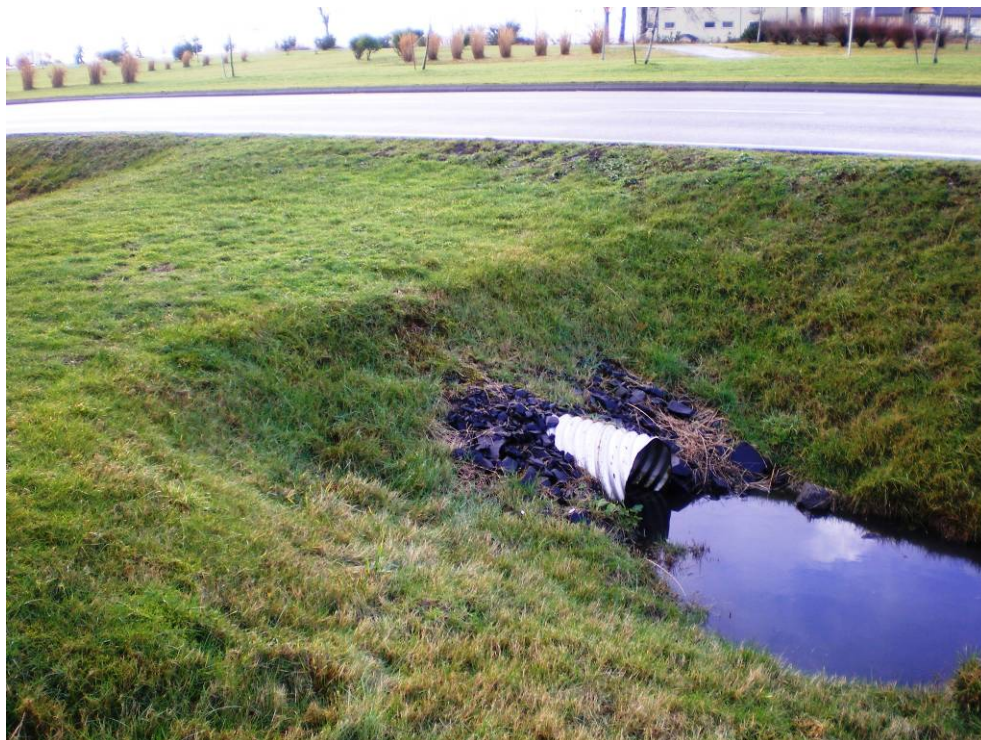
Photo 4: Swale outlet at the south end of the swale.
