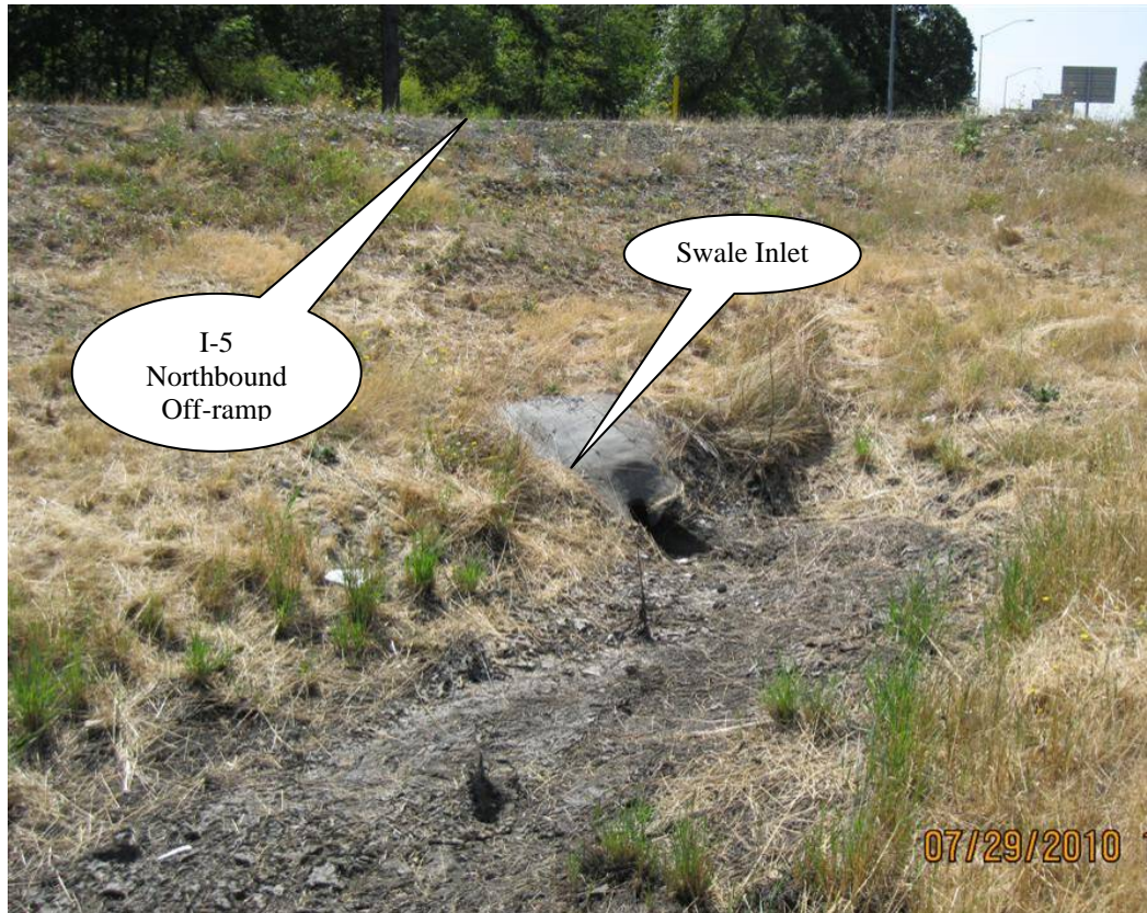
Photo 3: Swale inlet (looking south)
