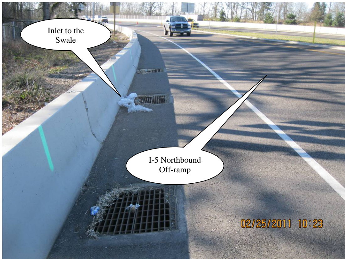
Photo 2: Inlets (looking south)
