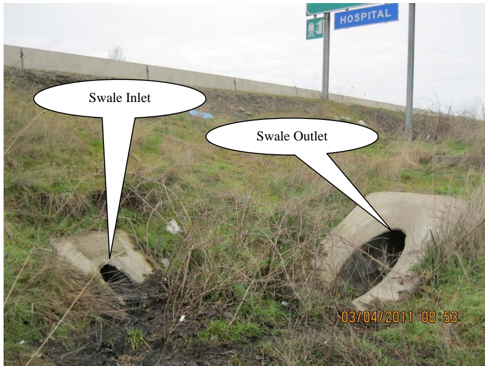
Photo 2: Inlet & Outlet of the Northern Swale.
