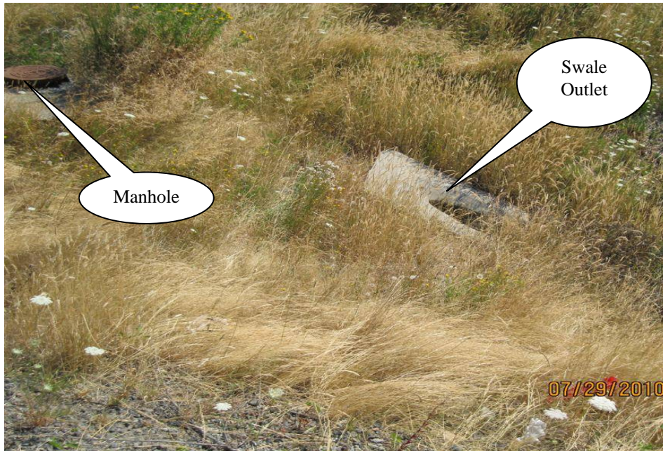
Photo 4: Outlet & Flow Control Manhole
