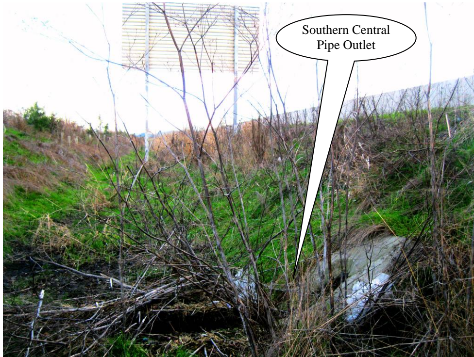
Photo 6: Southern central pipe outlet into swale (Point D on Operational Plans).
