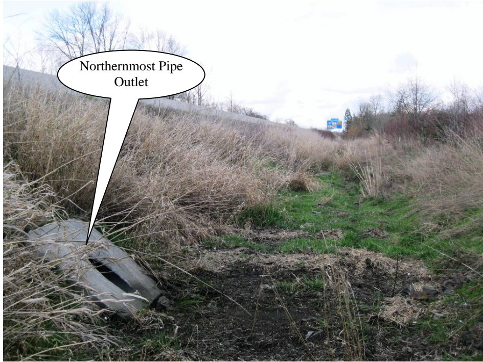
Photo 8: Northernmost pipe outlet into swale (Point F on Operational Plans..
