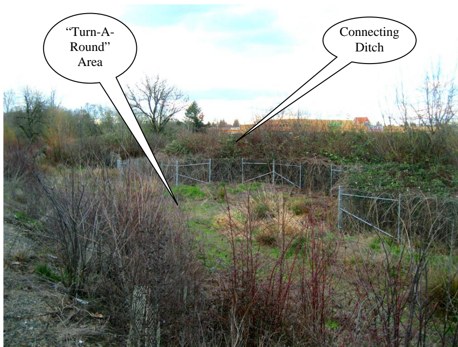
Photo 1: The ditch connecting Facility D00044 to Facility D00043 is behind a fence north of Facility D00044 (Point A on Operational Plan in Appendix A). A “Turn-A-Round” area is just west of the ditch and fence (Point B). This picture was taken facing northeast. D00044 is to the south of the pictured area and D00043 is to the north of the pictured area.
