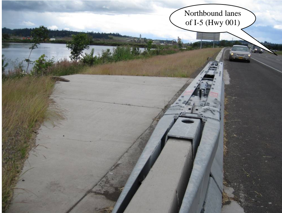
Photo 6: Swing gate at the southern end of adjoining facility D00044.
