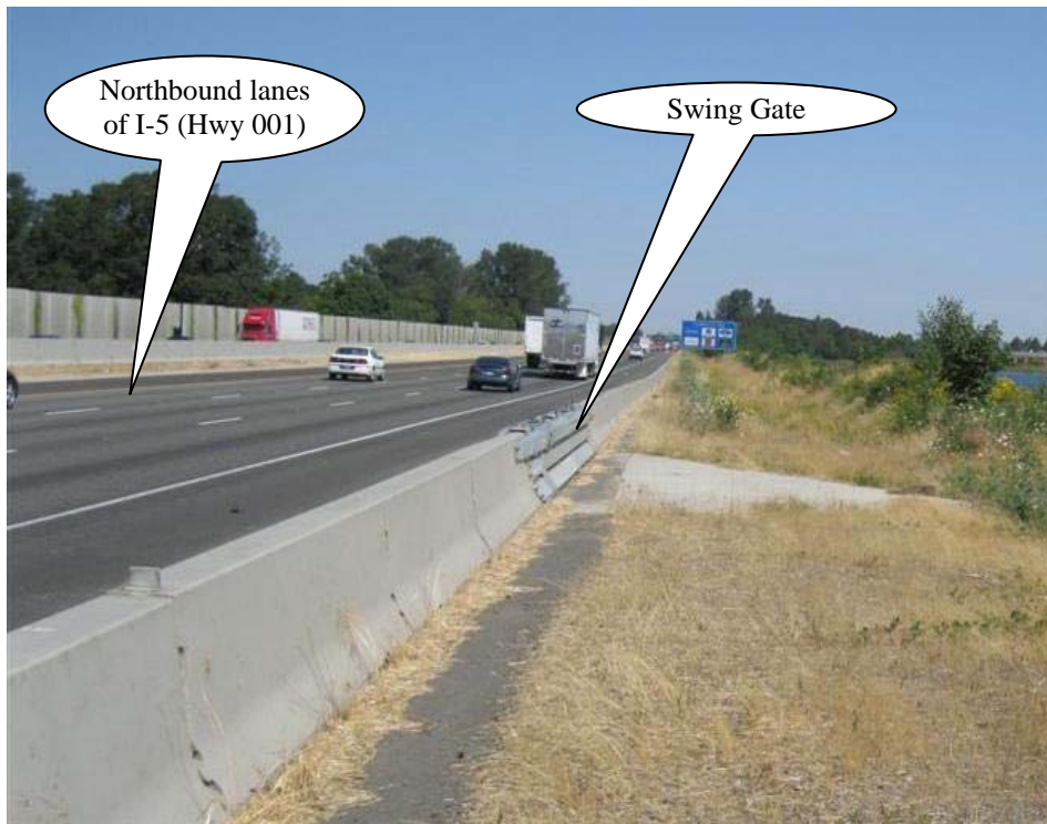
Photo 7: Swing gate at the southern end of adjoining facility D00044.
