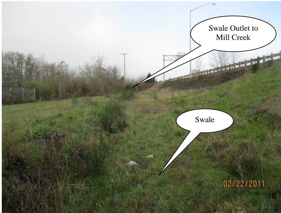
Photo 3: Swale channel and outlet, looking west.
