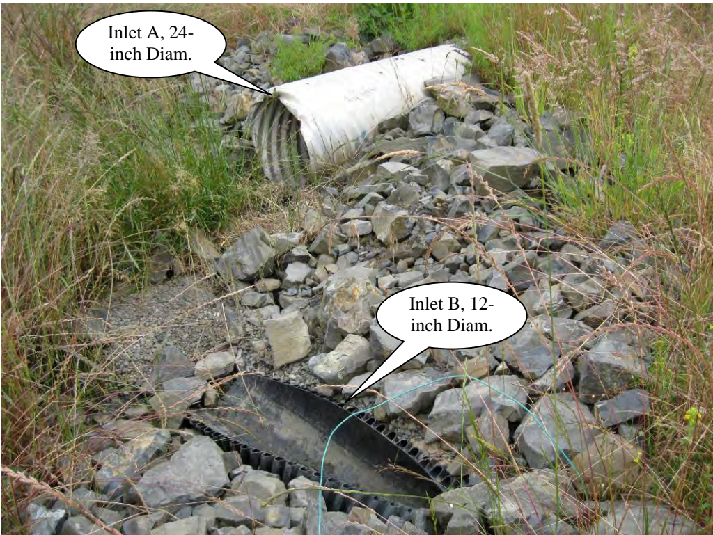
Photo 4: This photo shows the two facility inlets, Inlet A and Inlet B, at the south end of the facility. Flow spreader underneath formed of riprap. (Points A, B and C on the Operational Plan in Appendix A.)
