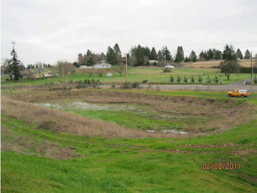
Photo 3: Vehicular maintenance access, which circles the pond/swale combo, is indicated by tire tracks.
