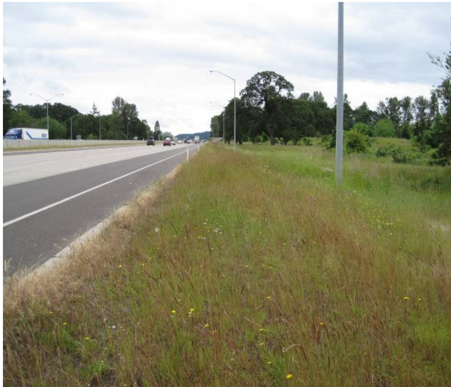
Photo 4: Access pond along I-5; (southbound lanes)
