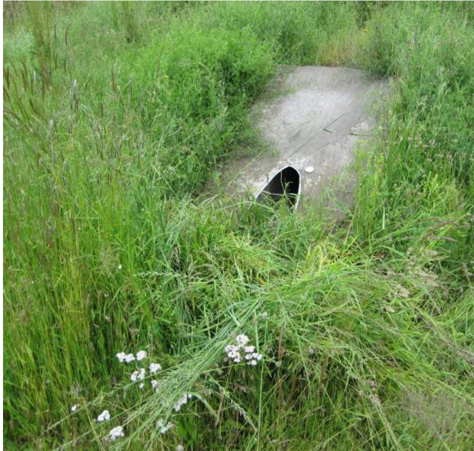
Photo 1: Pipe B is shown and drains runoff from Santiam Highway. All other pipe ends in the pond have a concrete collar.
