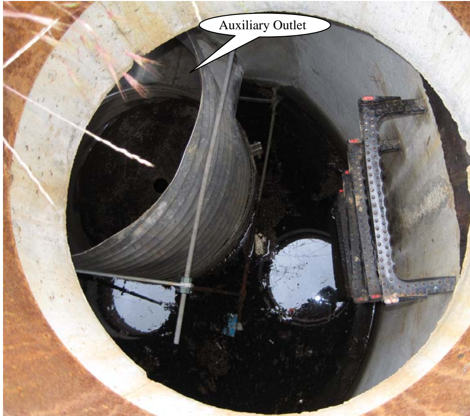
Photo 3: Flow control structure (Manhole interior)
