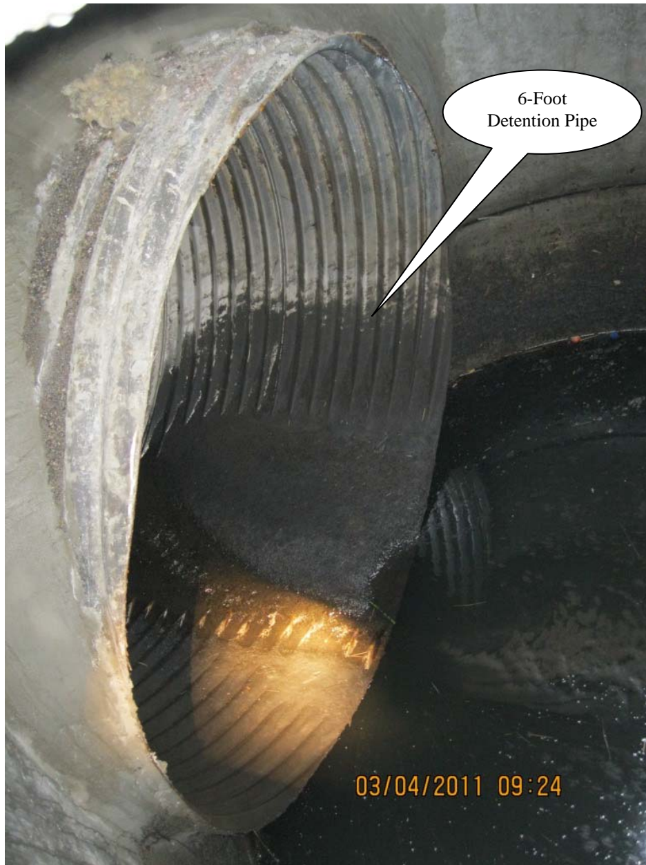
Photo 4: Detention Pipe (Point C, looking south)
