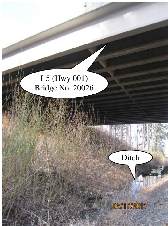
Photo 4: This ditch receives stormwater from D00038 as well as D00039 and D00034. (U.P.R.R railway to the right (north) not pictured.)
