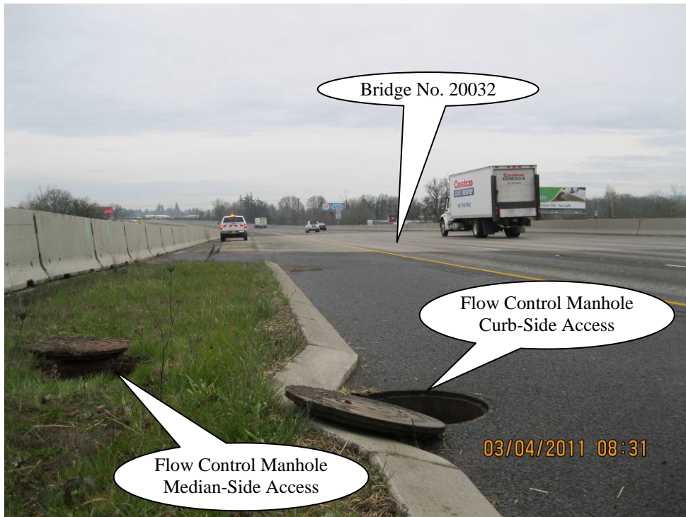
Photo 4: Drainage area. Photograph taken facing north.
