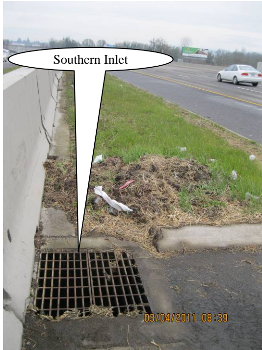
Photo 3: Southern inlet. The manhole attached to this inlet was not found during fieldwork, but it may exist. For the position of this manhole, refer to the Operational Plan in Appendix A and pages 16C and 16D in 38V-117 in Appendix B.
