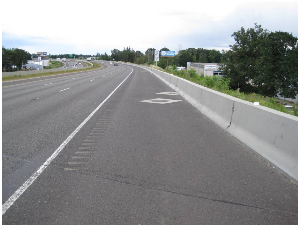
Photo 2: Detention pipe facility looking towards the north. This photo includes more of a view of I-5 northbound.
