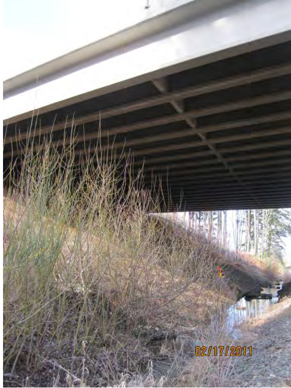
Photo 7: The drainage ditch receiving the water from the ditch inlet-outlet structure.
