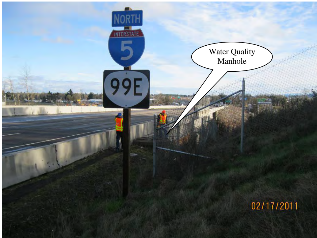
Photo 2: Water quality facility location with northbound travel lanes of I-5 (Hwy 001).
