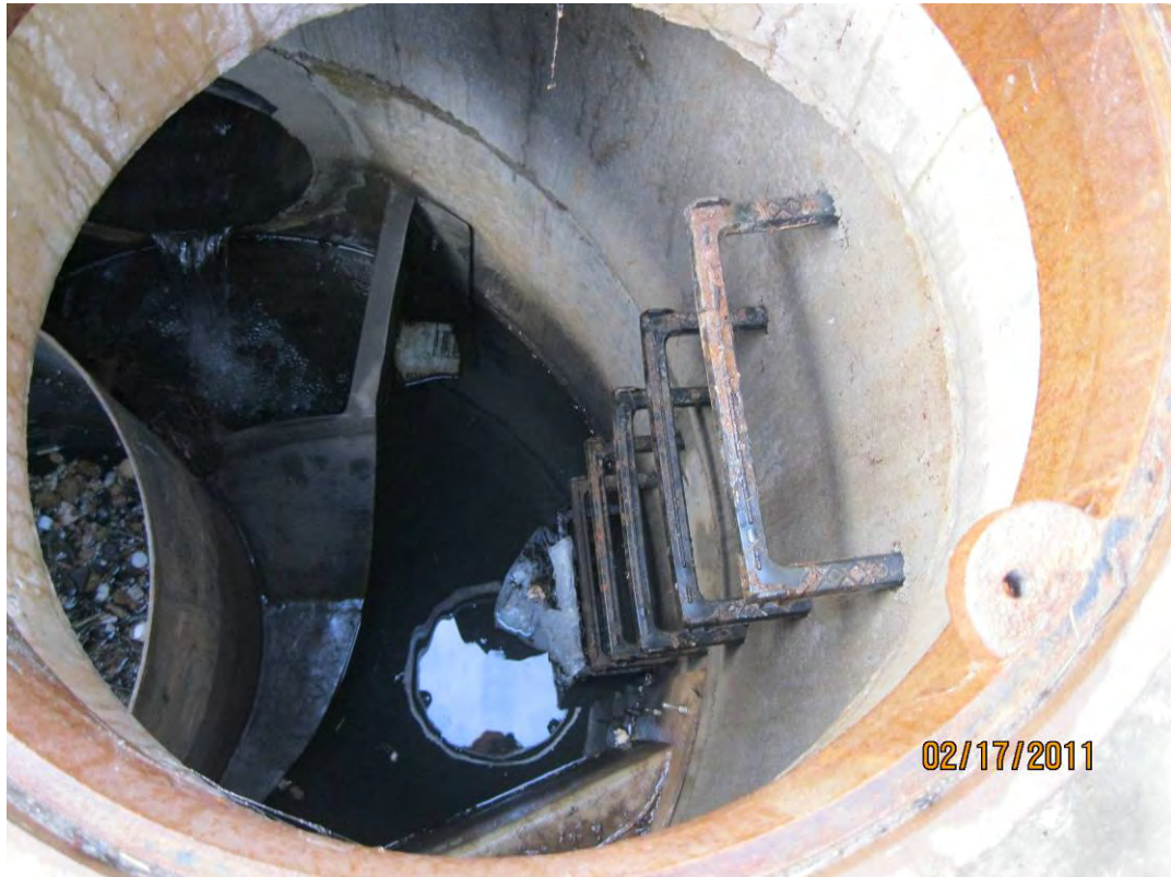
Photo 5: This photo depicts the access ladder for the facility.
