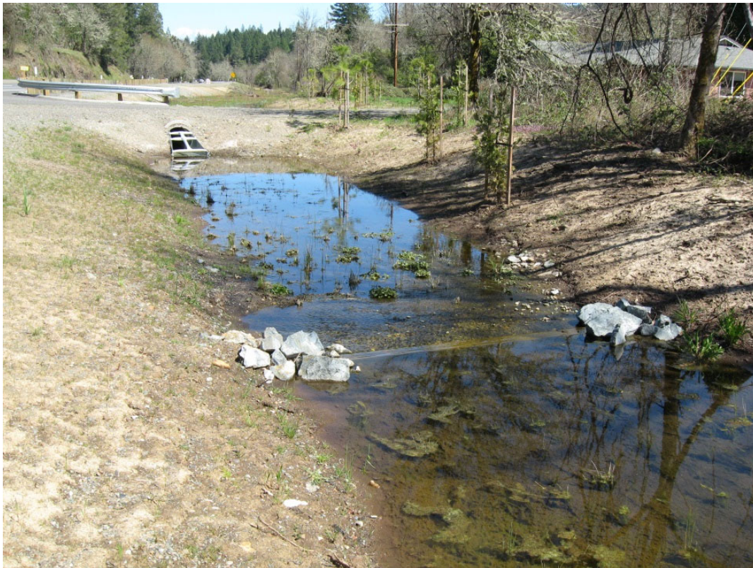
Figure 1: DFI No. D00002, looking north
