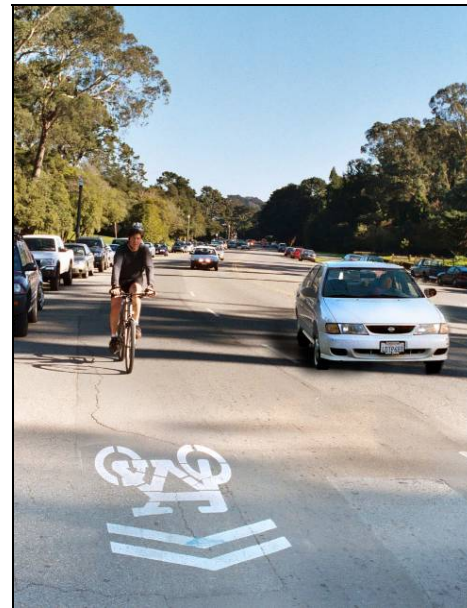
Figure 3.34: Shared Lane Markings Indicate Where a Bicyclist Should Ride in the Roadway
