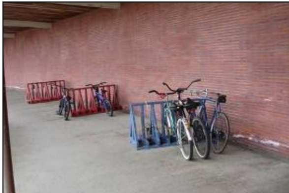
Figure 26: Poorly Designed Bike Racks at Seaside High School
