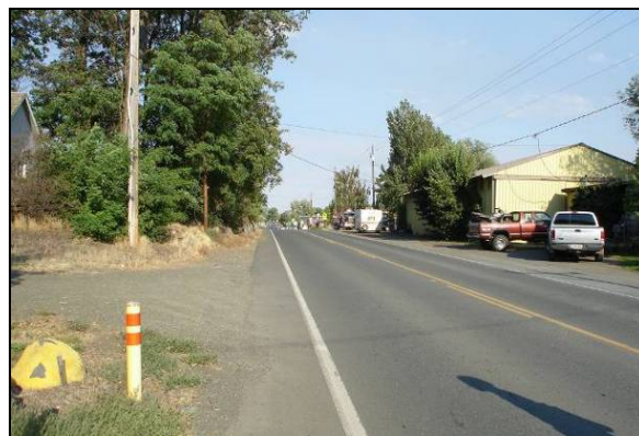
Figure 3.25: Shoulder Bikeways Are Appropriate Along Wide Roads Where Vehicles can Avoid Passing Close to Bicyclists
