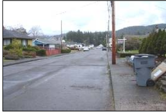
Figure 16: 17th Avenue Sidewalk with Reduced Pedestrian Zone due to Presence of Power Pole and Trash Can
