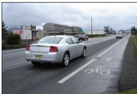
Figure 27: US 101 Bike Lane with Gravel and Debris Stretching down the Middle of the Lane – will Require Bicyclist to Ride too far Inside Near Pavement Edge or Far outside Near Moving Vehicles
