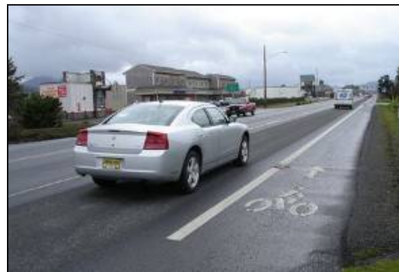
Figure 3.33: US 101 Existing Bike Lane
