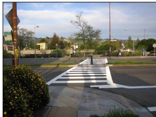
Figure 3.29: High-visibility Crossings Are Well Marked with Crosswalk Striping, and Can Include Signage and Pedestrian Refuge Islands
