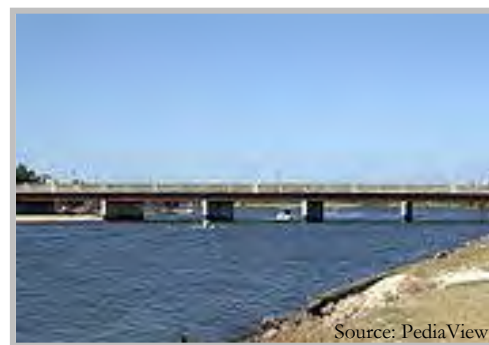
Example of causeway built on piers
