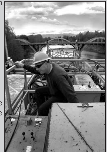
7th Street Bridge work
