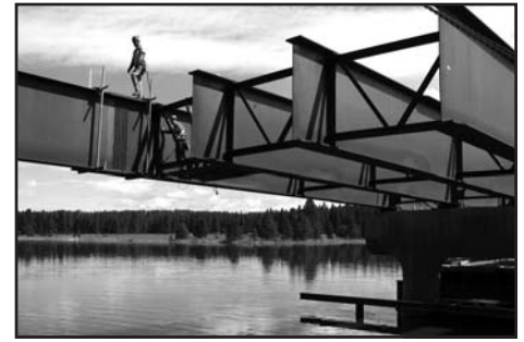
Spencer Creek Bridge
