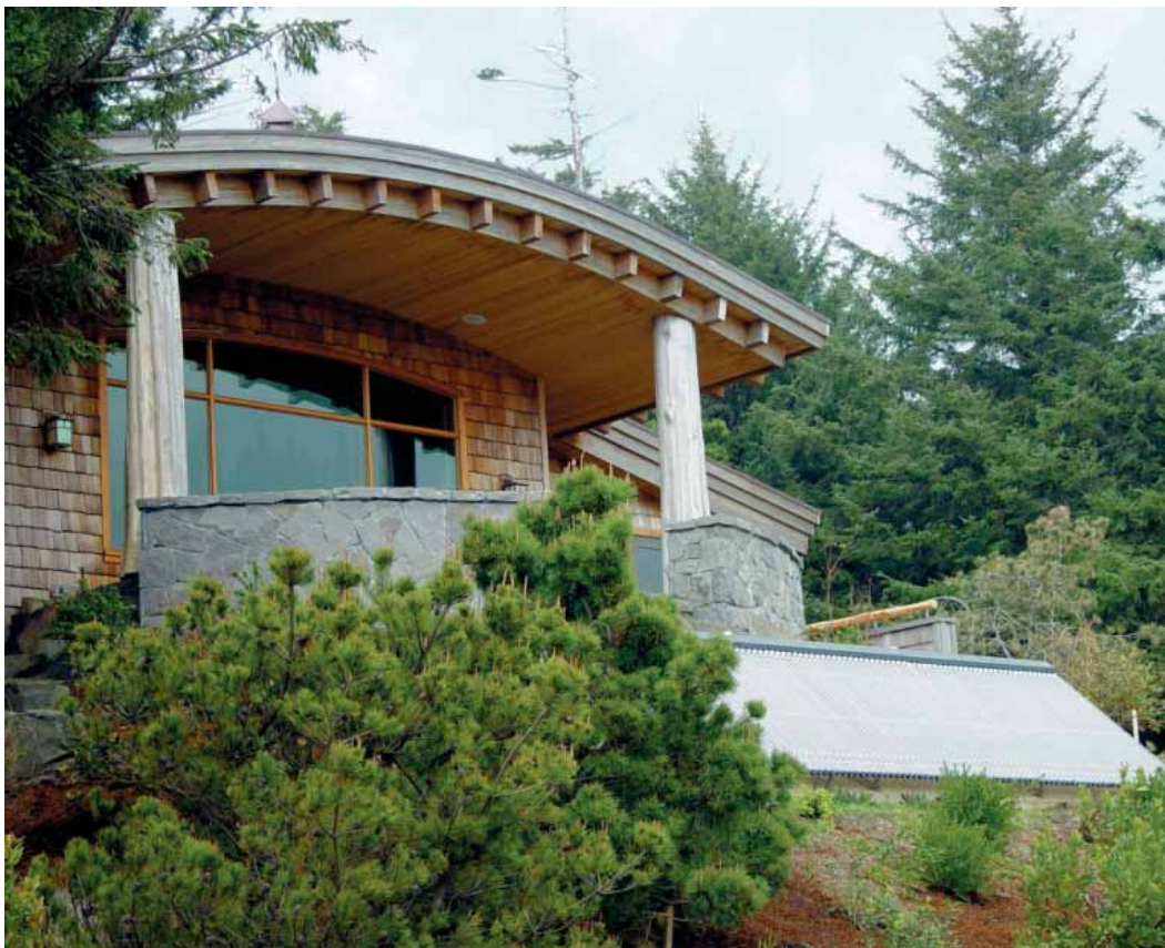
Left: The 90 Thermomax® evacuated tube solar collectors are placed on the embankment below the front patio.
