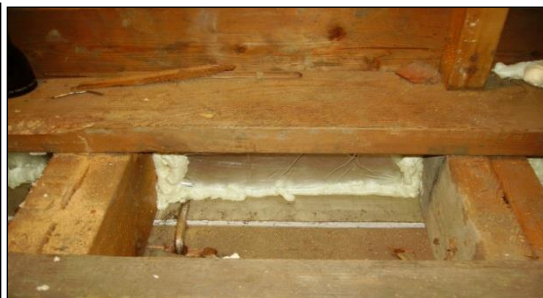
Knee wall blocks needed before insulating
