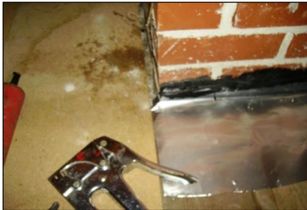
Sealing of a chimney chase way
