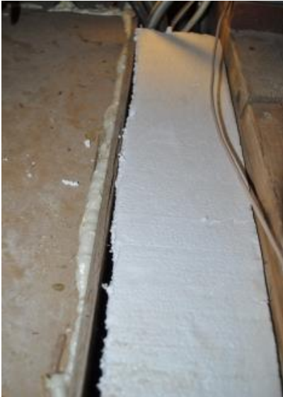
After capping, chases must be sealed
