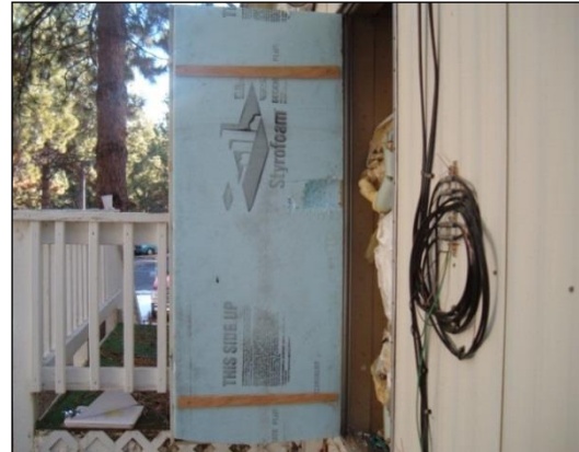
Water heater closet door insulated with foam board
