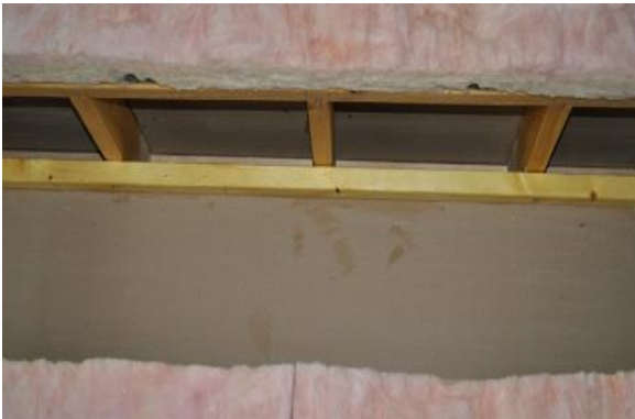
Clear work area of insulation and debris.
