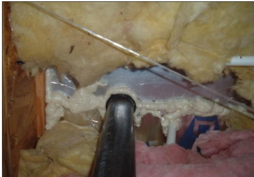
Plumbing penetration sealed
