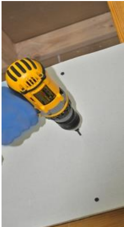
Bracing can be screwed to drywall before capping the chase
