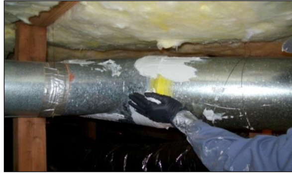
Mastic Being Applied Over Mesh Tape
