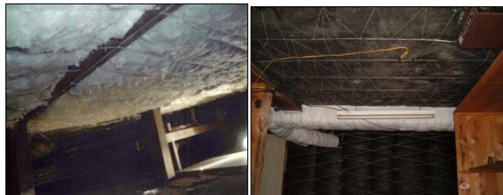
Twining under site built floors
