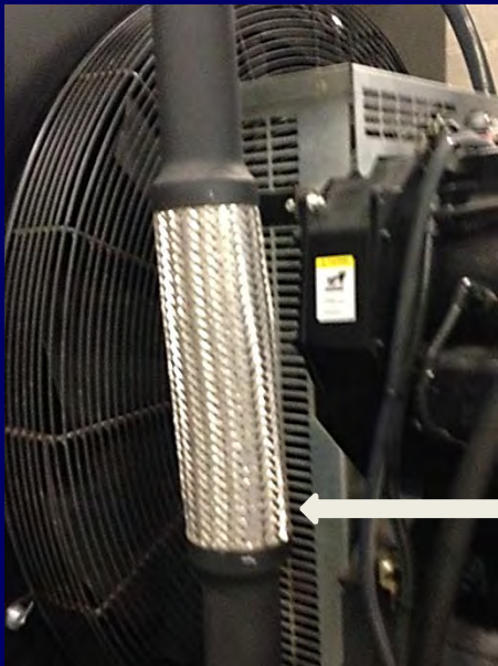
Flexible Connections
