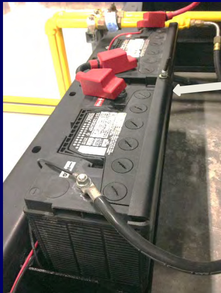
Strapped Batteries
