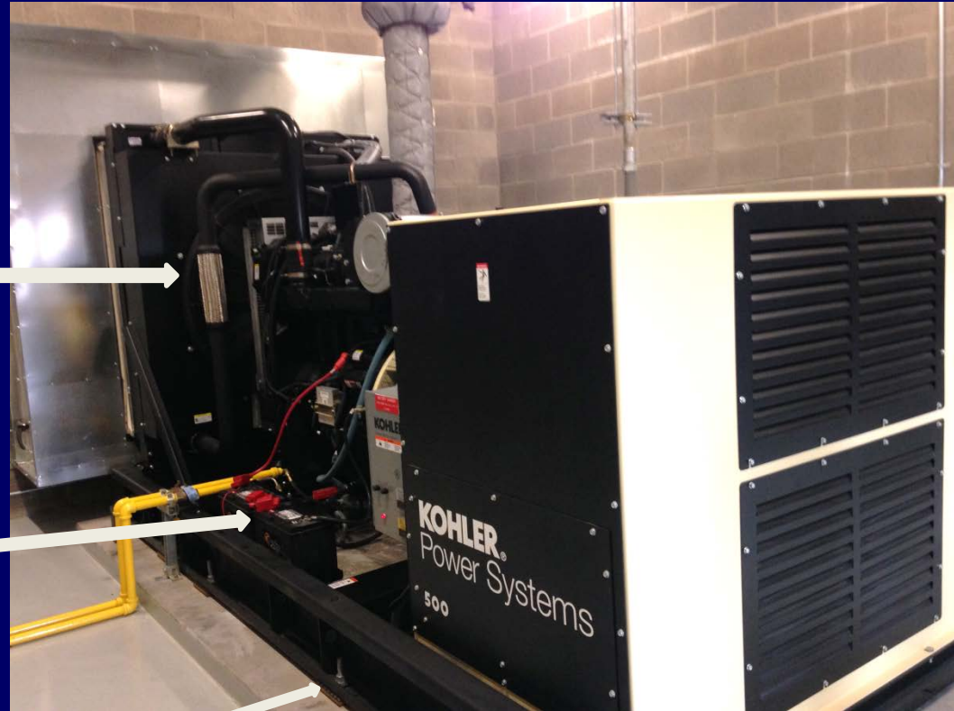
Anchored for earthquake shaking
