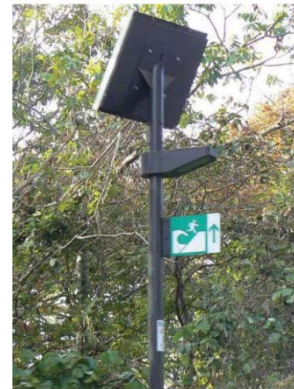
Figure 4. Use of solar panels help to illuminate signs during night time.
