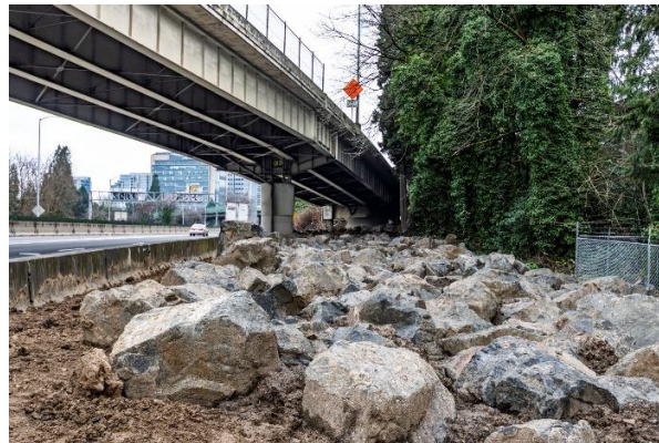
Photo: Oregon Department of Transportation
