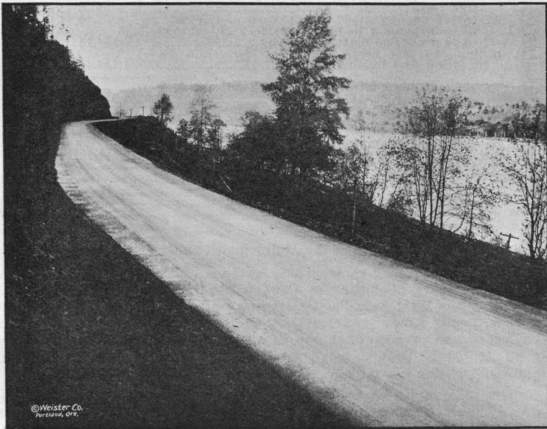
BITUMINOUS PAVEMENT ON THE PACIFIC HIGHWAY SOUTH OF OREGON CITY IN CLACKAMAS COUNTY. GRADED AND PAVED IN 1918
