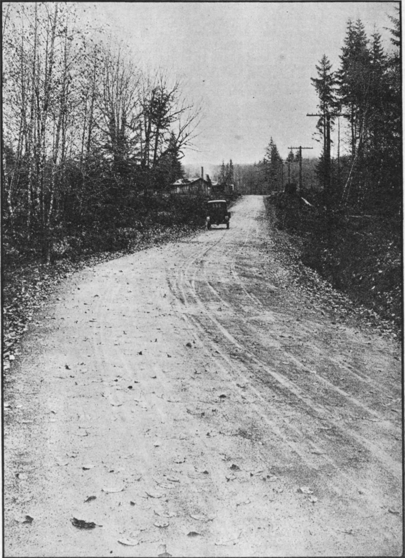
BITUMINOUS PAVING NEAR SVENSON IN CLATSOP COUNTY ON THE COLUMBIA RIVER HIGHWAY. PAVED IN 1917
