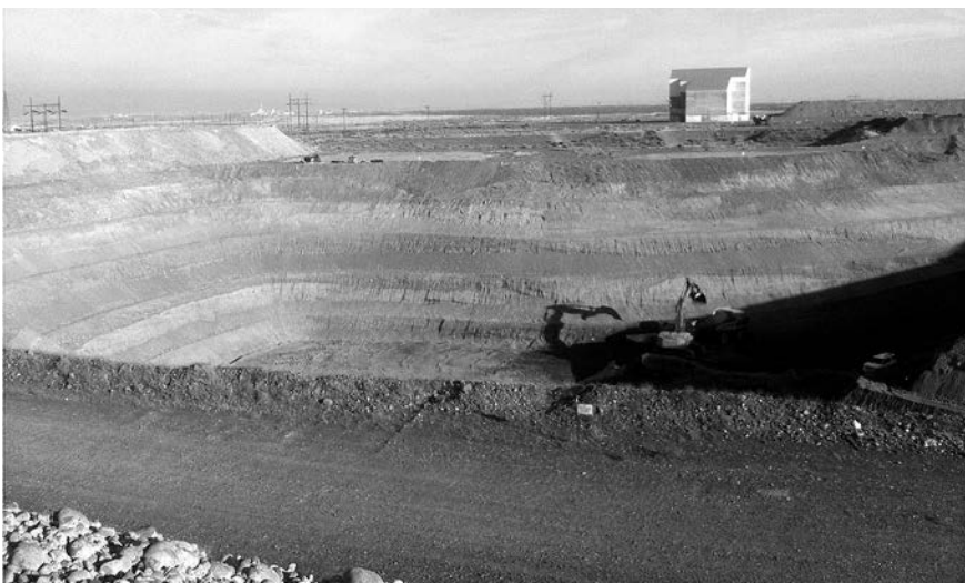
◀ Hanford workers dug to groundwater near C Reactor in pursuit of a plume of Hexavalent chromium.
