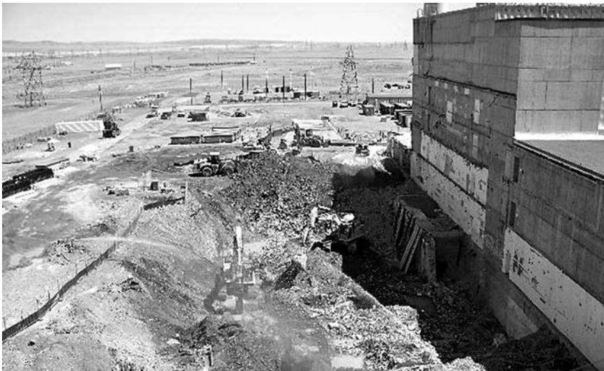
◀ Excavation work next to the K-East Reactor.
