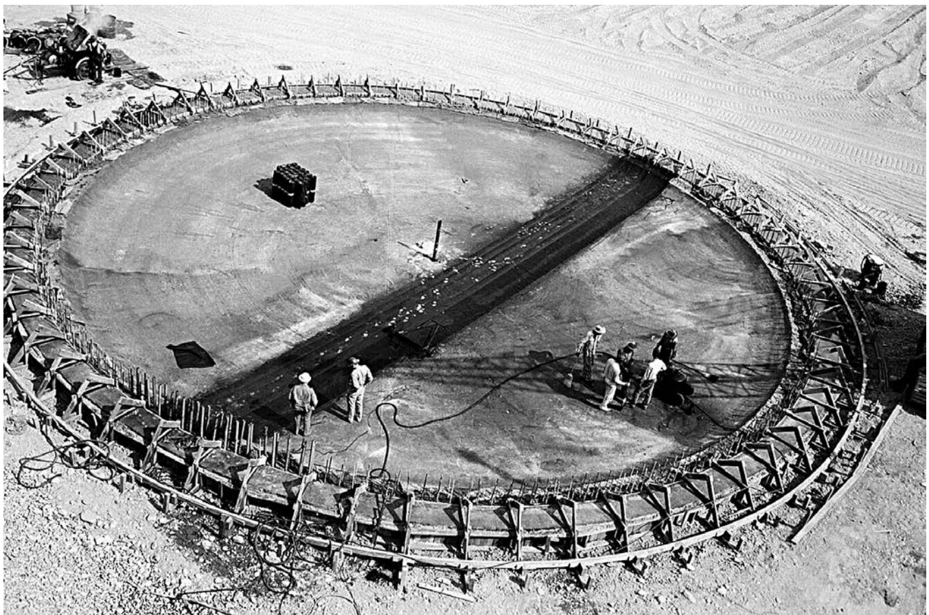
Construction of Hanford’s BX Tank Farm, March 1947. ▼
