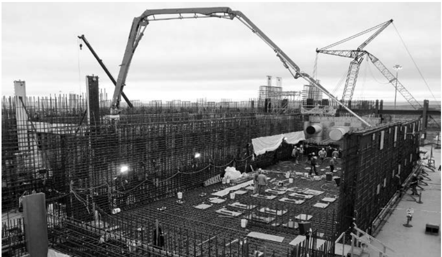
Construction work at Hanford's Waste Treatment Plant. ►
