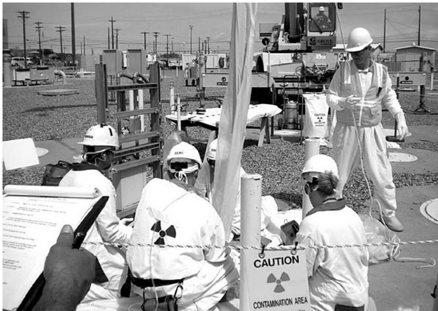
◀ Workers in a Hanford tank farm.
