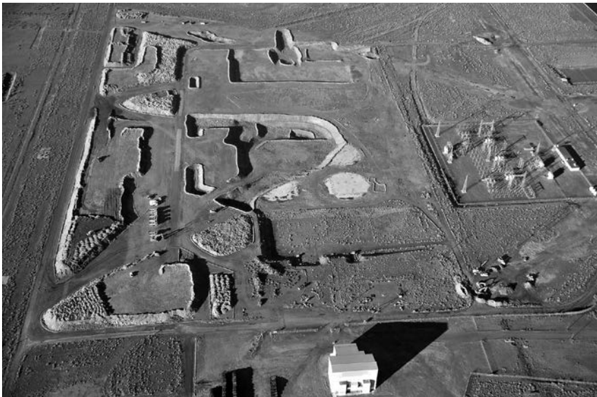
◀ Workers dug a large pit near the cocooned C Reactor in pursuit of Hexavalent chromium (and later dug a second large pit as well).
