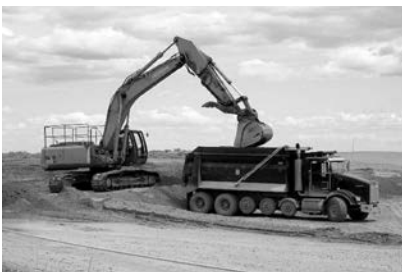
▲ Contaminated soil is loaded in the BC Control Area.
