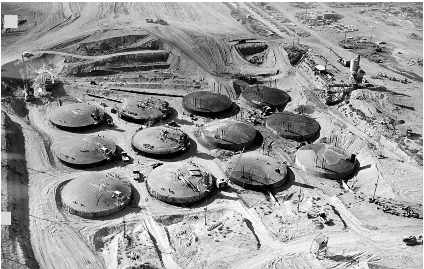
▼ Hanford tanks under construction.
