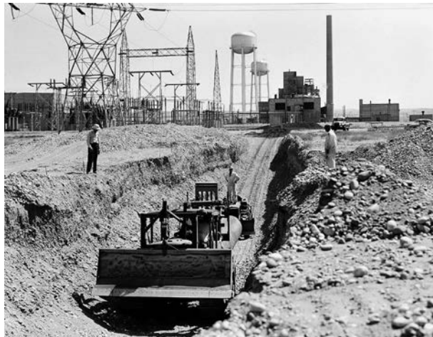
Construction of a burial ground in Hanford’s 200 West Area.
