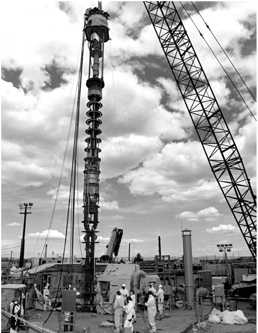
Installing mixer pump in tank SY-101. ►
