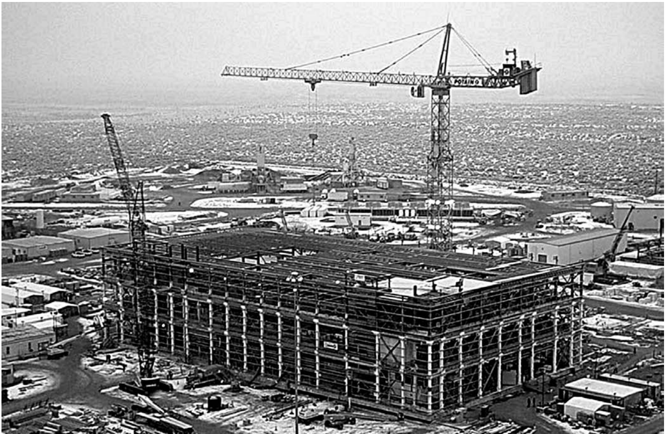
▲ The Waste Treatment Plant's Low-Activity Waste Vitrification facility, December 2005.
