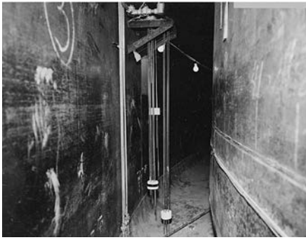
▲ The annulus of tank AY-102 during construction.
