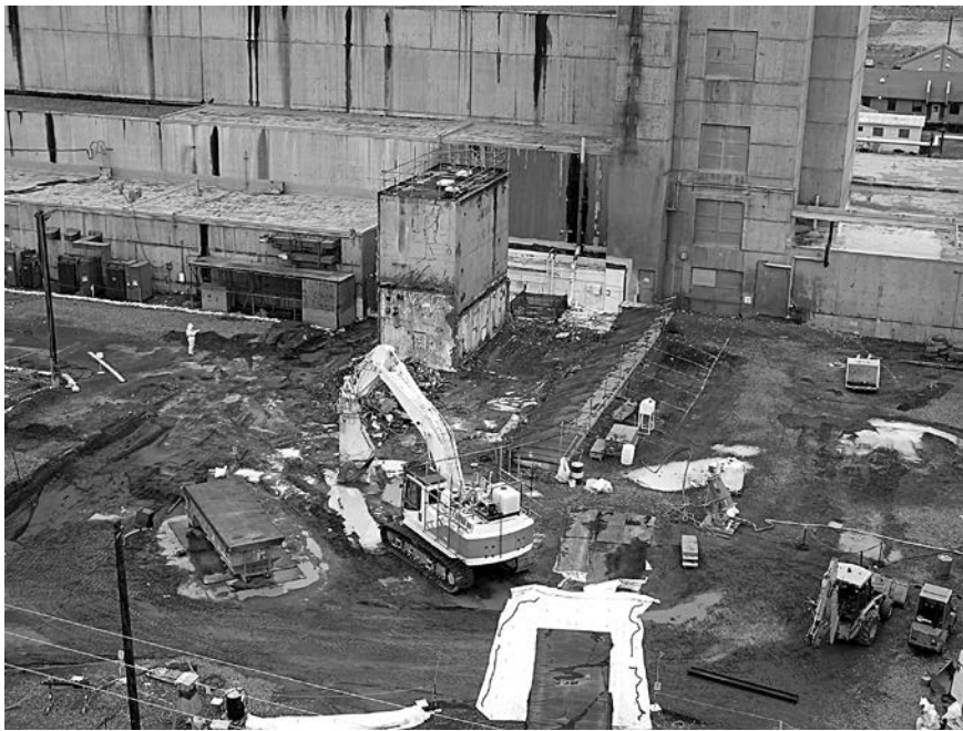
◀ Demolition work on the 233-S facility.
