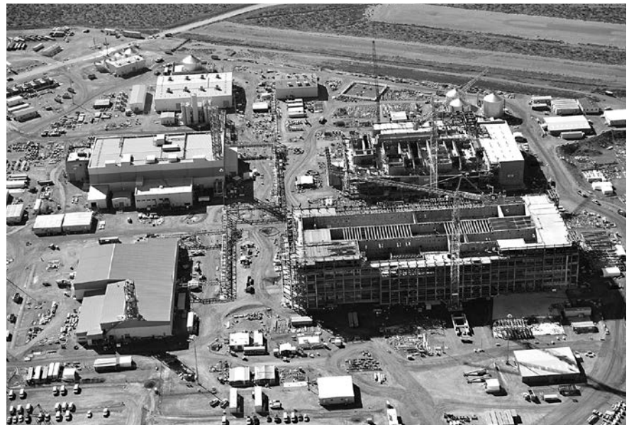
Aerial of the Waste Treatment Plant. ▶
