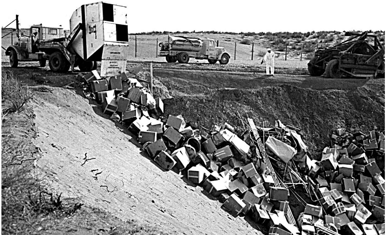
Waste being dumped into a 300 Area burial ground in 1955. ▼
