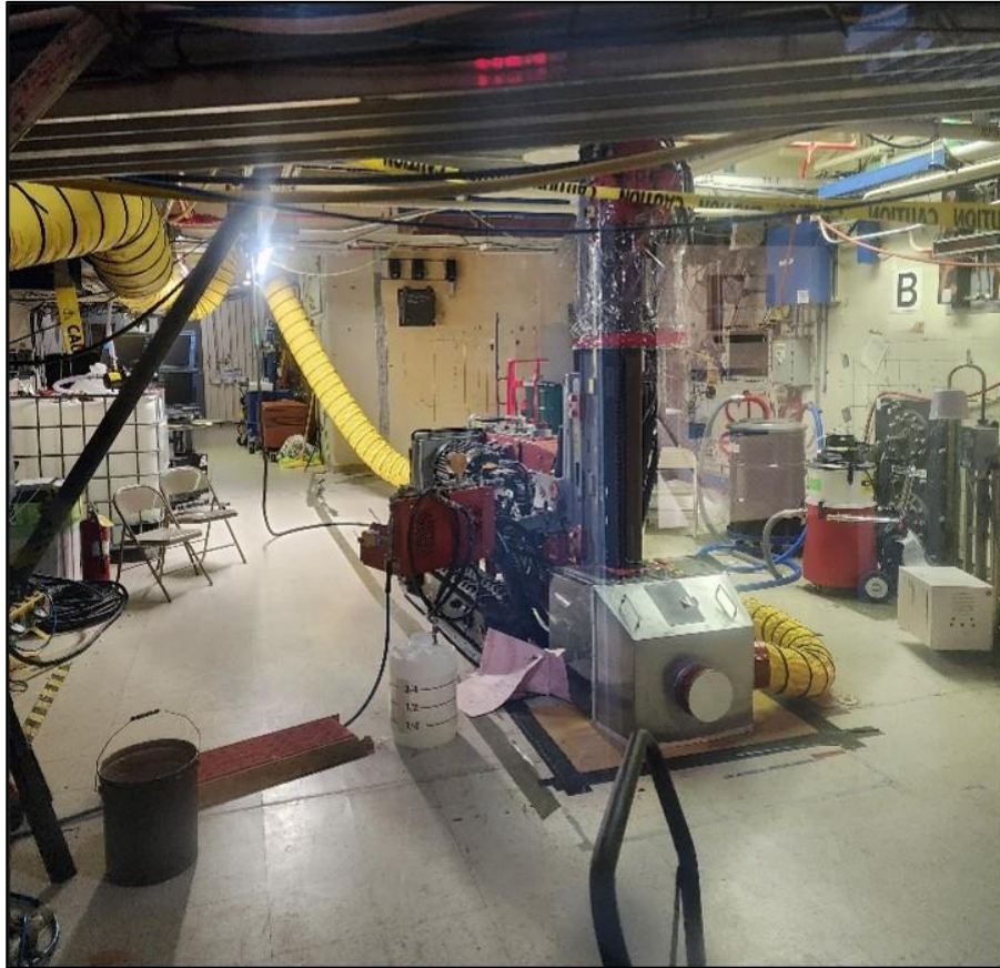
A drill in room 131 of the 324 Building supports vertical soil-stabilization work.
